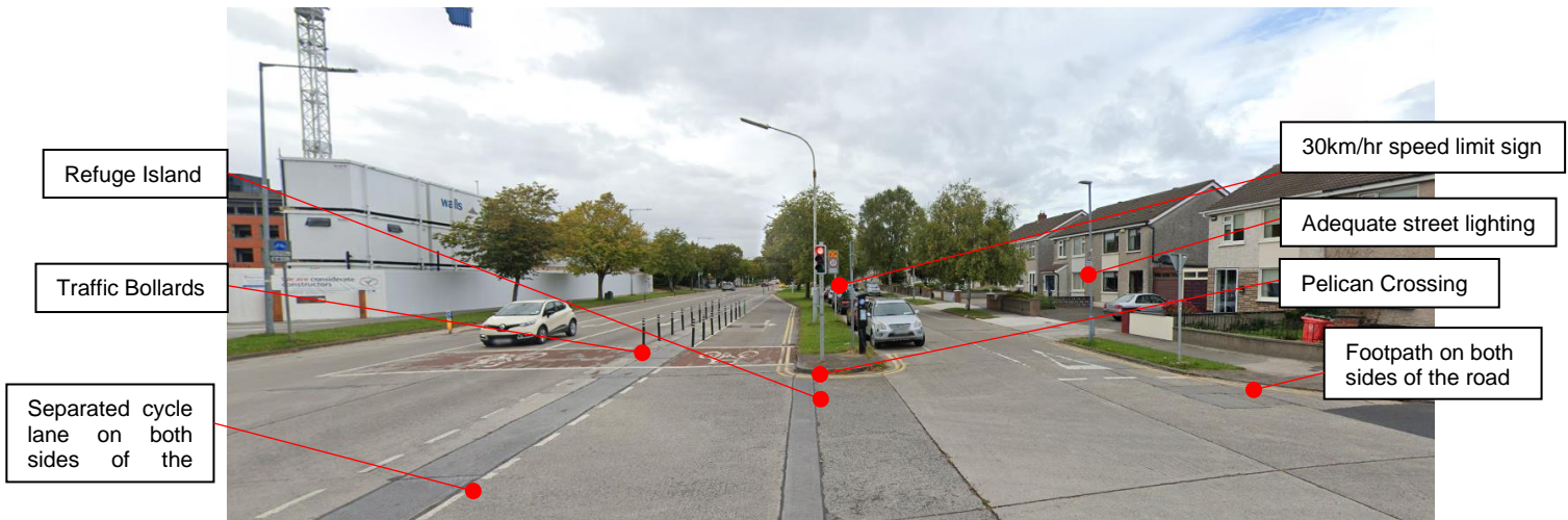
Figure 4-3 – R103 street view towards the R108
