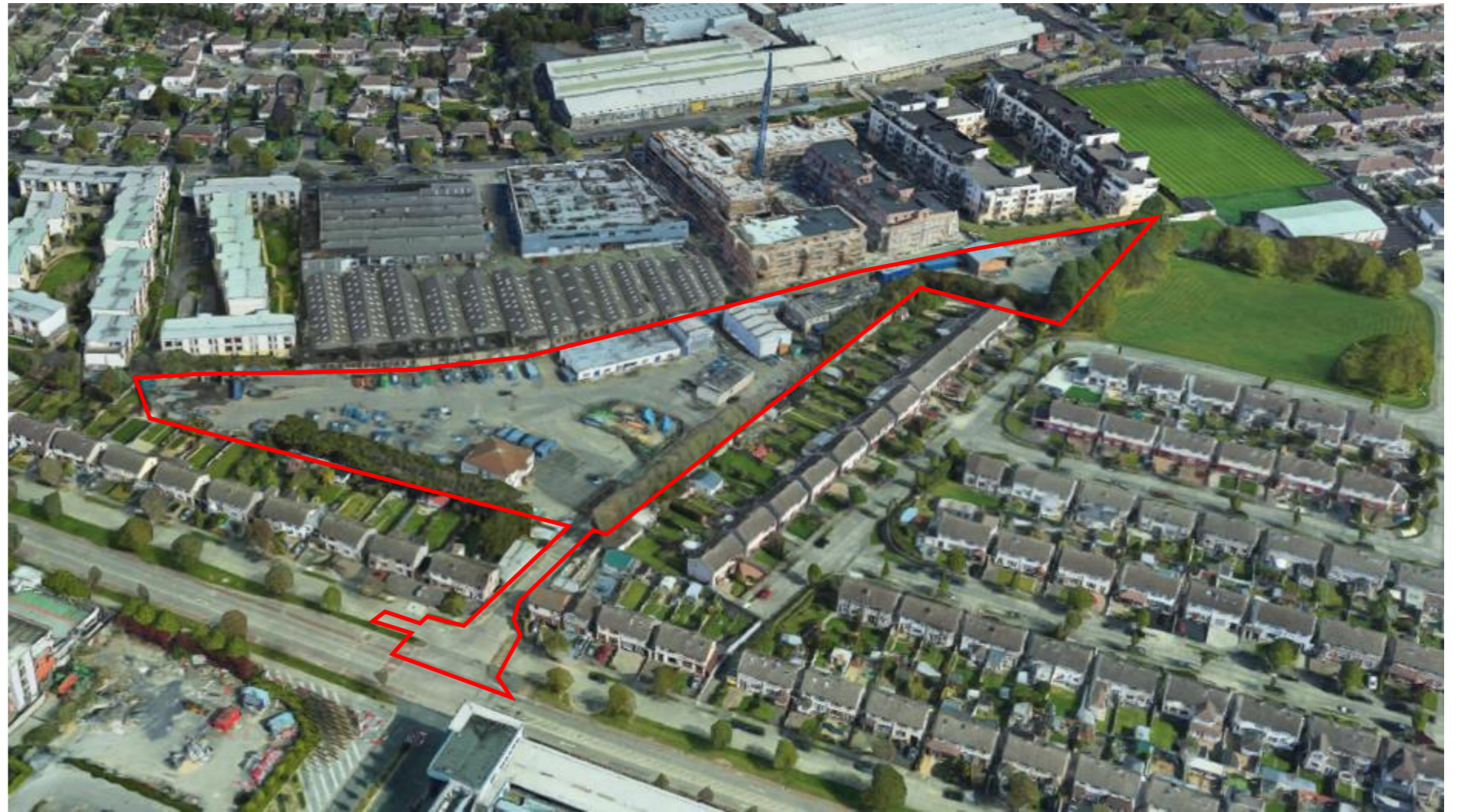
Figure 5: birds eye view of site with proposed application boundary outlined in red
