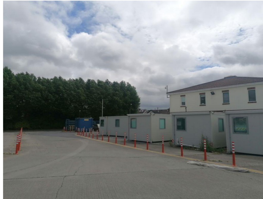
Figure 17: view of existing administration building and temporary structures
