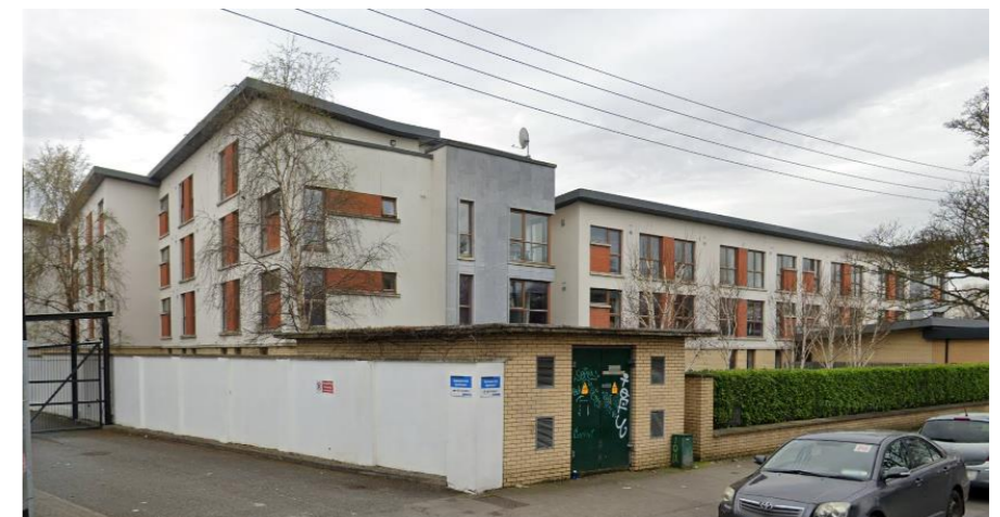
Figure 15: existing view of Shanowen Hall
