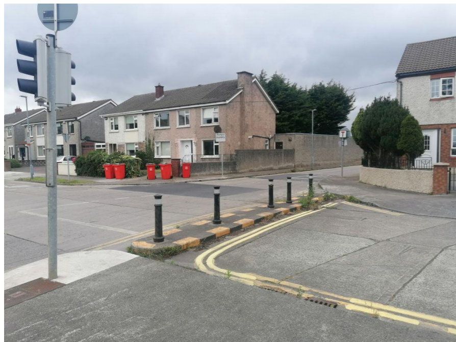
Figure 4: view of existing entrance junction at Collins Avenue
