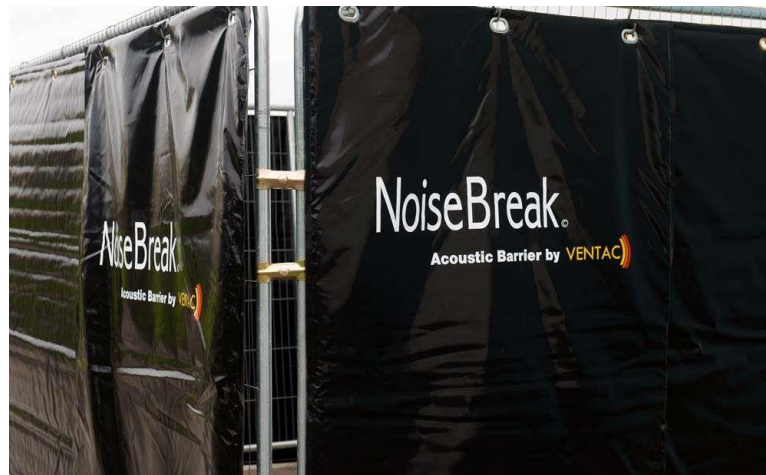
Figure 14: Temporary Construction Noise Barrier © Ventac
