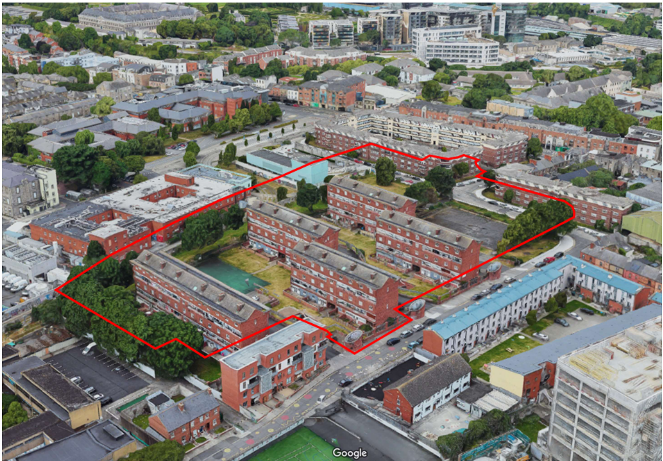
Figure 3: Aerial View of the Existing Site Layout
