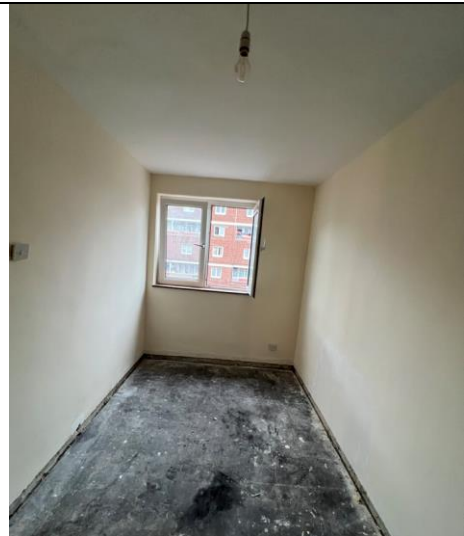
External wall- Internal view- Photo 14
