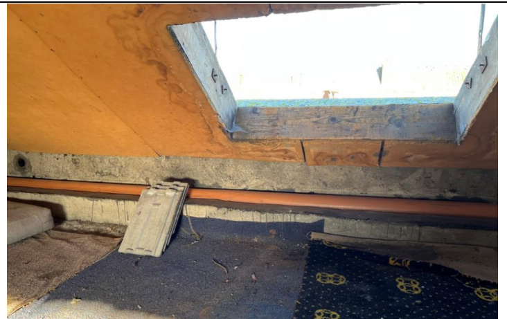
Attic structure- Internal view- Photo 12
