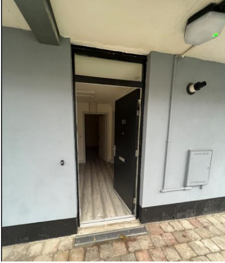
Ground Floor apartment - Photo 1
