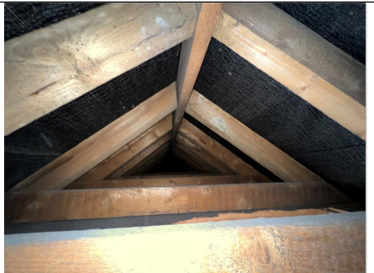
Attic structure- Internal view- Photo 10
