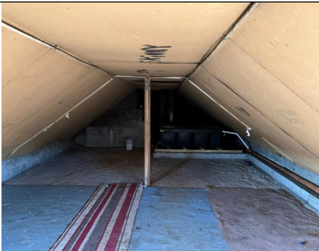
Attic - Internal view- Photo 9
