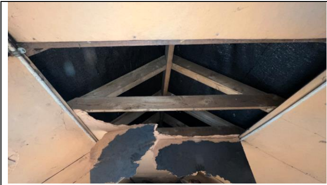
Attic structure- Internal view- Photo 11
