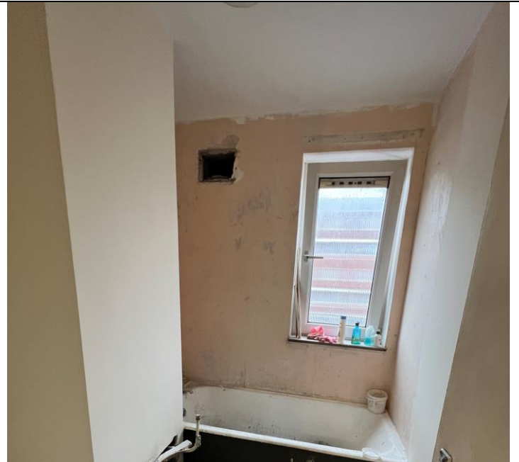
External wall- Internal view- Photo 16
