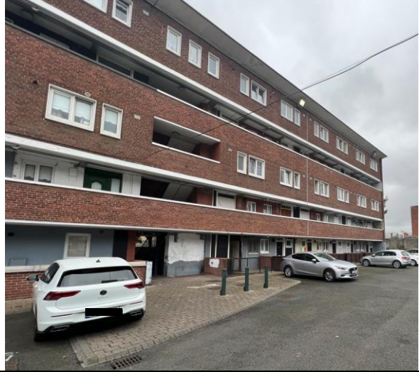
Ground Floor - external side - Photo 2
