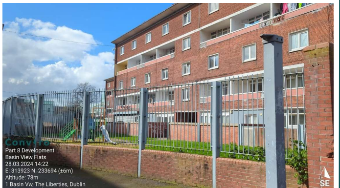
Photo 4: Existing residential flats requiring demolition.
