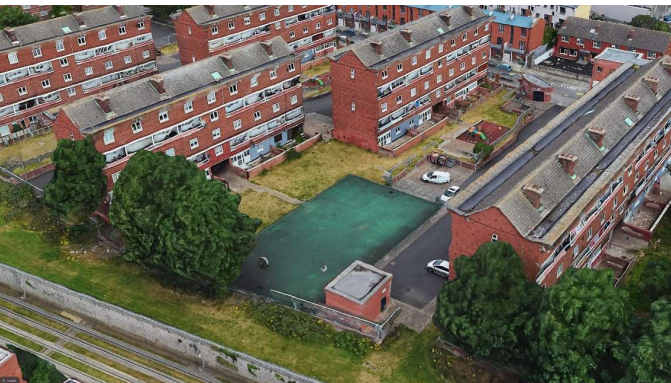
Photo 7: Existing play areas and structures requiring demolition (Ref. Google Earth).
