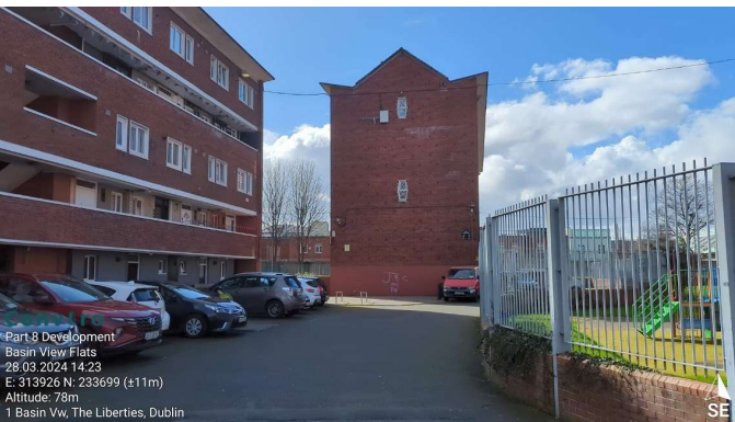
Photo 5: Existing residential flats requiring demolition..
