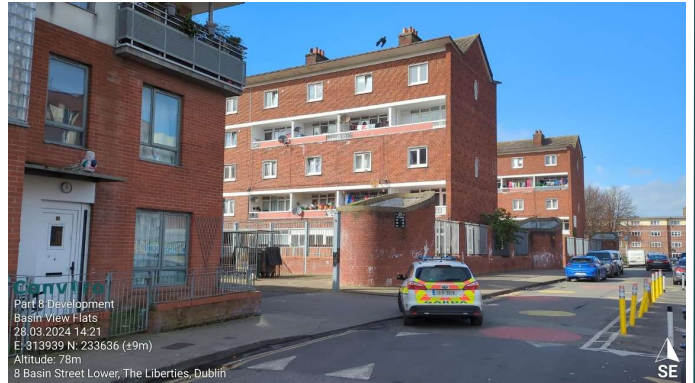
Photo 2: Existing residential flats requiring demolition.
