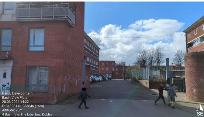
Photo 3: Existing tarmac surfaces requiring removal.
