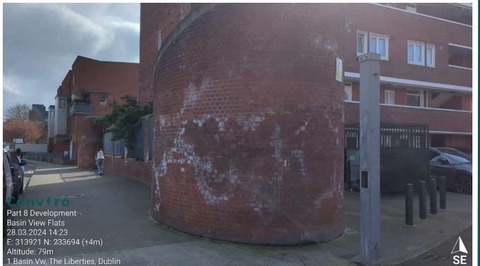
Photo 6: Existing structures requiring demolition
