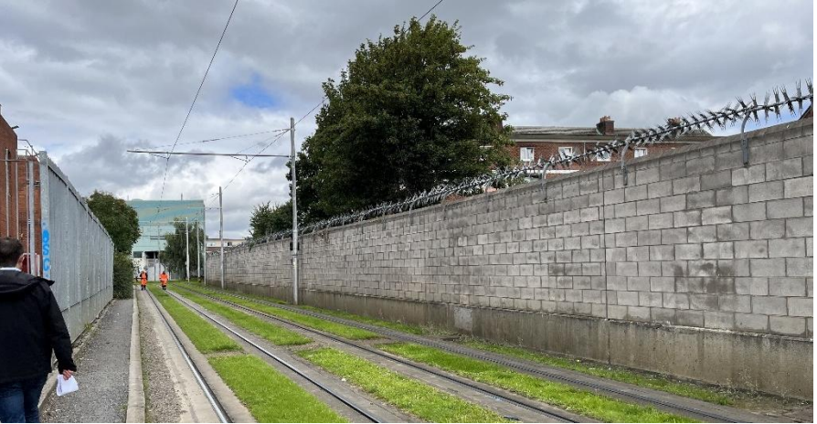
Figure 9: view down Luas tracks along western boundary towards mortuary building
