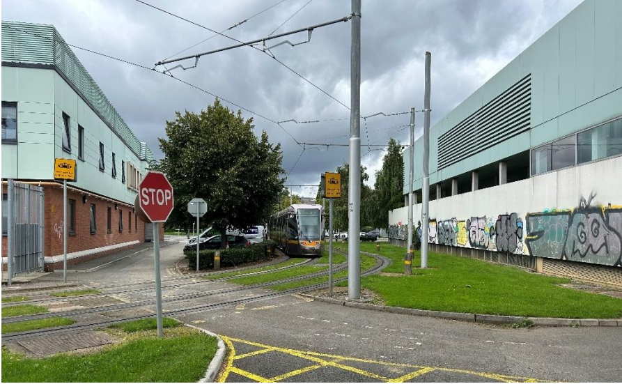
Figure 12: view of Luas tracks at St James's Hospital Mortuary
