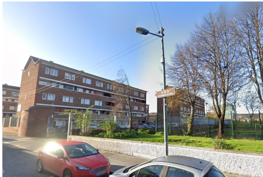
Figure 42: view of existing Blocks 1&2 and Oisín Kelly Park
