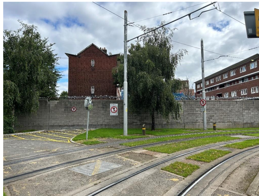
Figure 26: existing boundary to Luas line.
