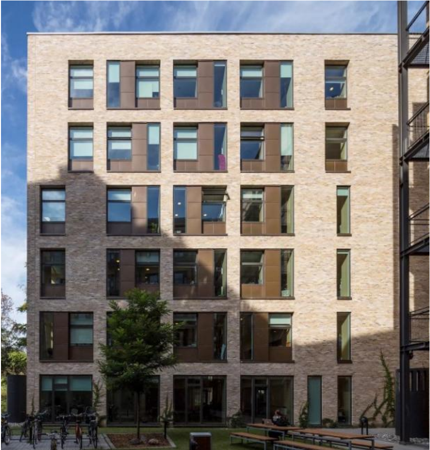
Figure 80: Reference image- buff brick and aluminium cladding
