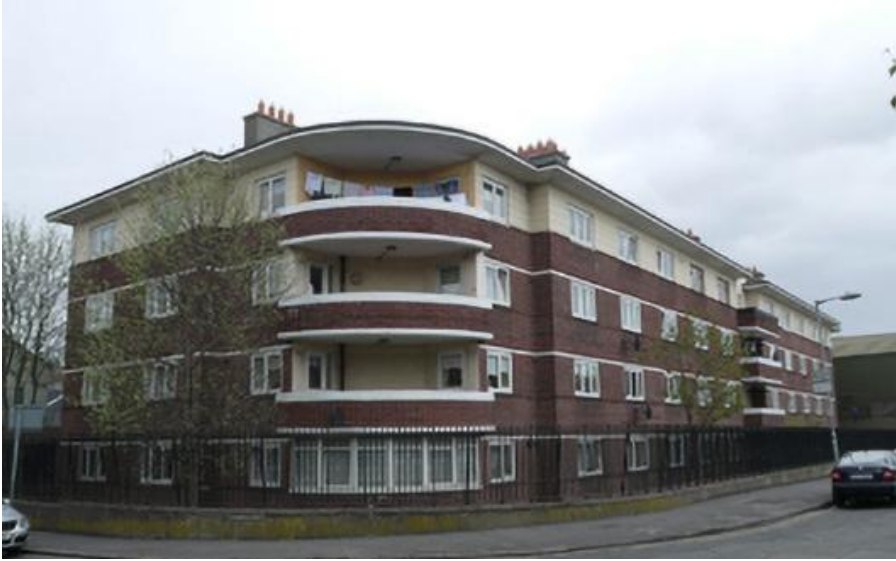
Figure 5: view of Mary Aikenhead House Flats on Basin Street Lower
