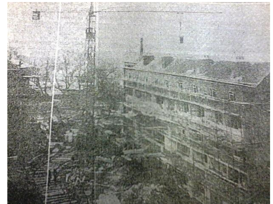
Figure 19: Basin View Flats under construction.
