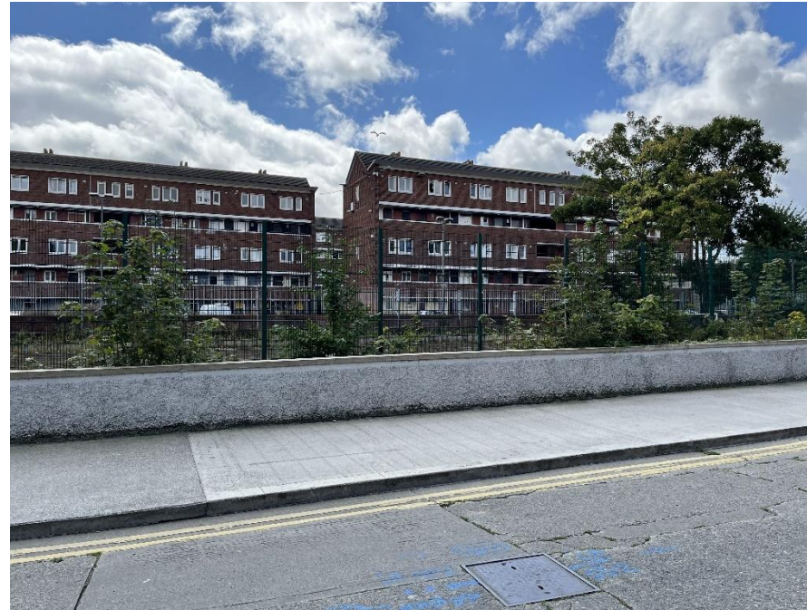
Figure 25: existing boundary to Oisín Kelly Park on Basin Street Lower
