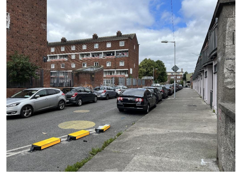
Figure 27: existing boundary to Brandon Terrace.
