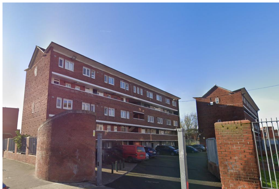
Figure 43: view of existing Blocks 3&4
