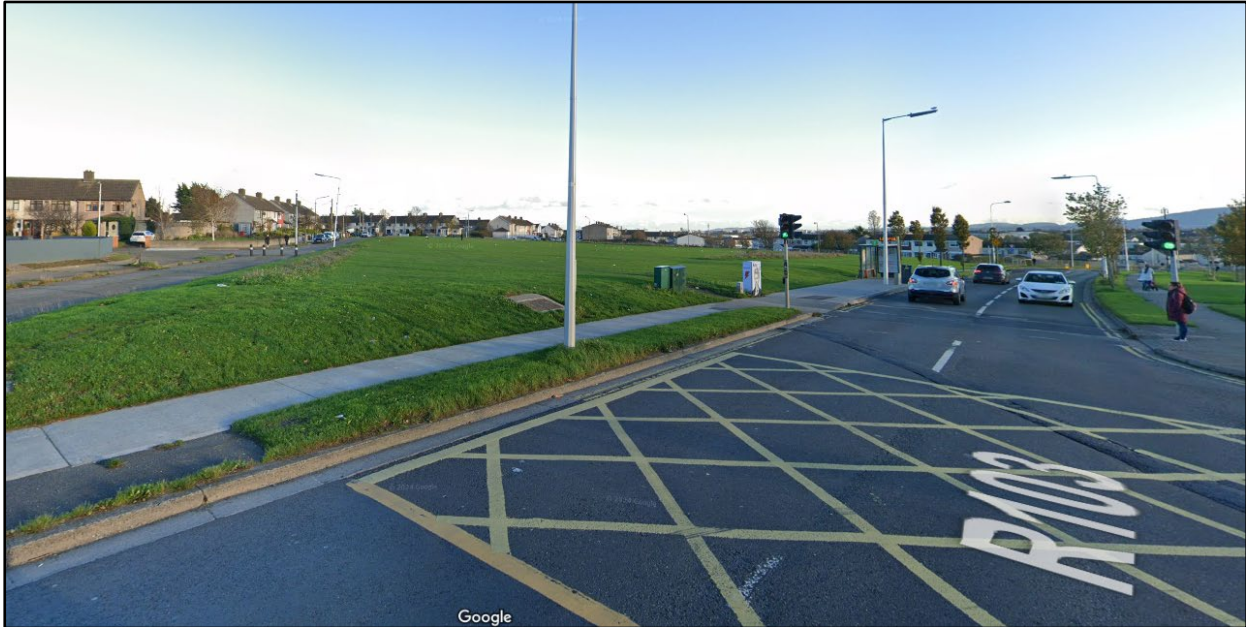
Figure 5.1a: Site access point northeast of site boundary (Source: Google Maps).
