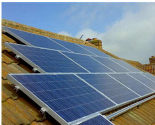
Typical Photovoltaic Arrangement
