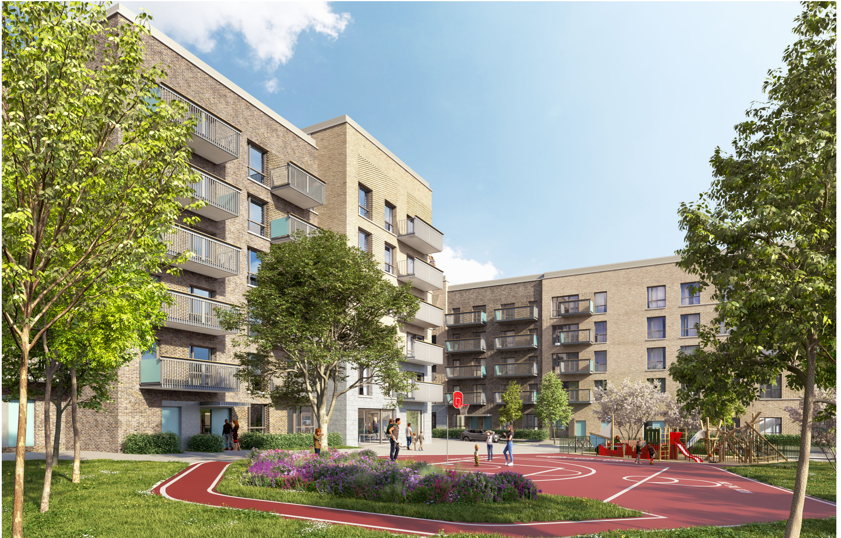
Above: View from Public Open Space looking east
