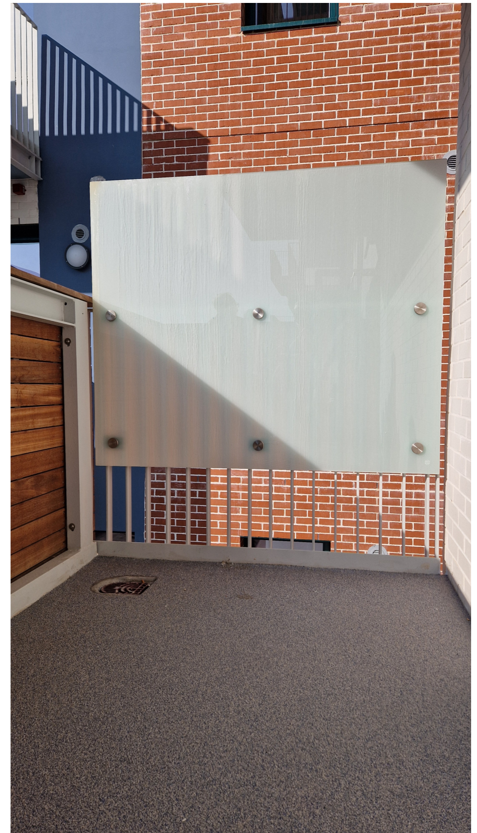
Above: Opaque glazed screen providing privacy between adjacent balconies
