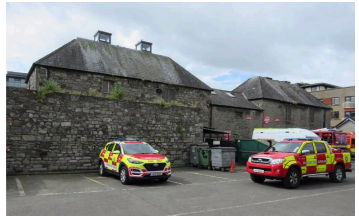
Above: View of the north façade of the Maltings from the subject site. The proposed development will respect this adjacent protected structure, and will provide a conservation gain in providing access for a greater audience to this visual amenity
