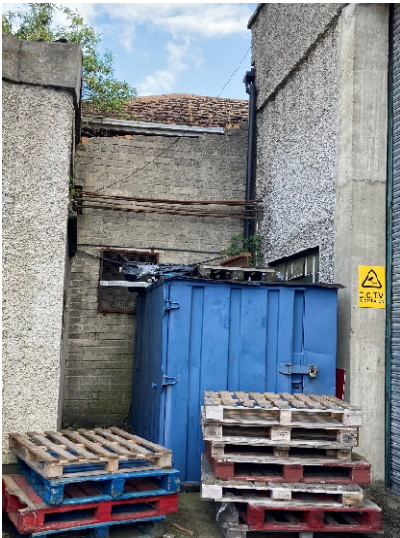
Figure 4.9 Solid Blockwork wall of 200mm Thickness
