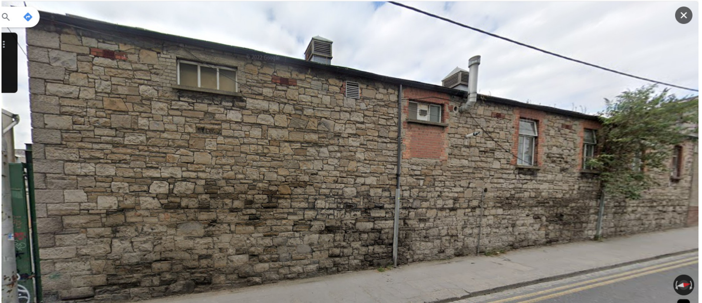
Figure 4.5 (500mm wide stone walls, upper ground floor)
