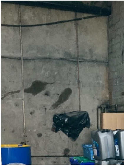
Figure 4.10 Internal photos-oil store
