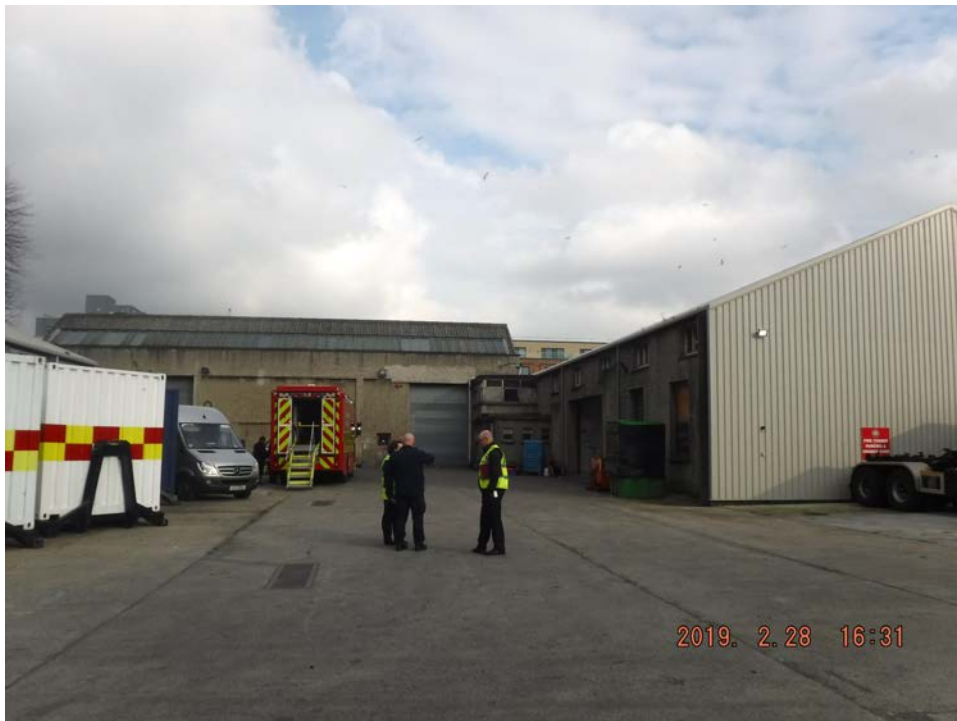
Plate No. 30. General view looking east showing the same early 20 th century two storey range of stores in 2019, after the demolition of the five storey block that was shown in the previous photo. The structure in the distance to the left, is a large concrete framed storage shed that has an entrance from Grangegorman Lower, and was shown on the 1972 Ordnance Survey map.
