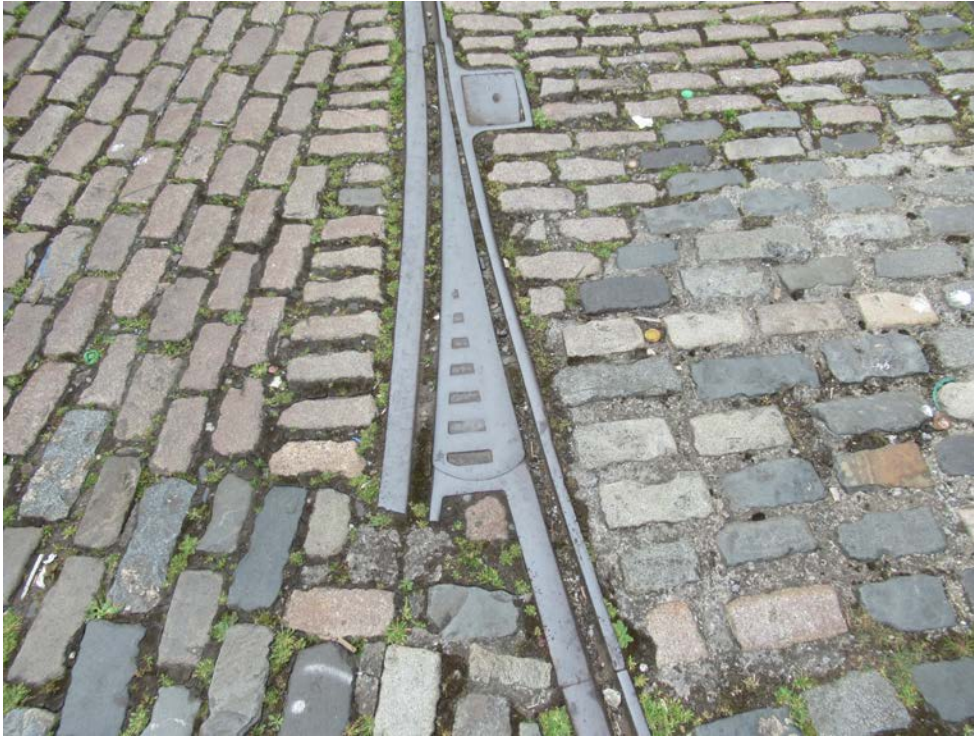
Plate No. 14. Detail view showing the early 20 th century tram track and colourful paving setts in the north end of Stanley Street. The section of poorly laid setts at the right of the photo are evidence of a poorly crafted repair to the paving. It appears that the setts have been placed on their sides instead with on their edges, and setts from different sources have been introduced that are of different colours and sizes.
