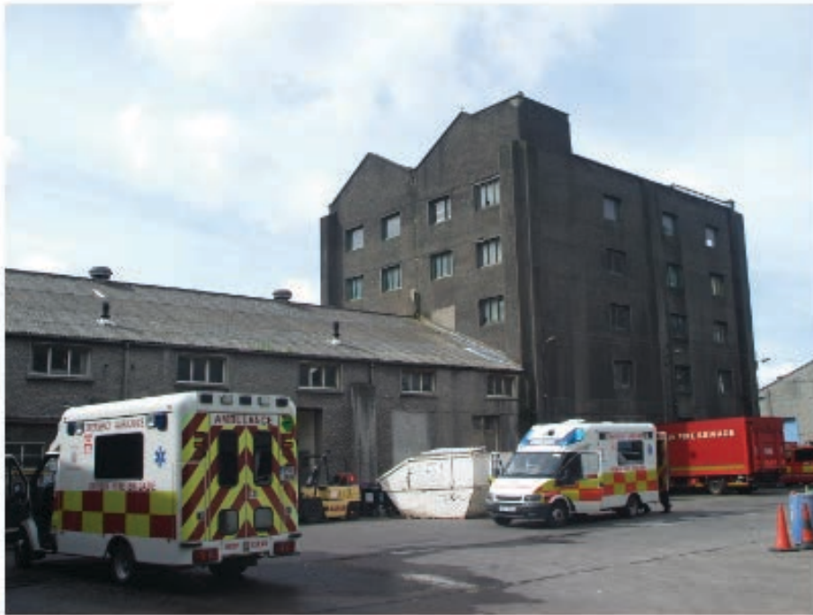
Plate No. 29. General view looking south-west around 2008, showing the long narrow two storey range along the north side of the central block of garages, along with its original early 20 th century five-storey western block, later demolished around 2010-2015. No trace of this structure currently survives on the site.
