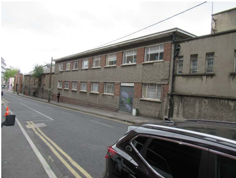
Plate No. 23. General view looking west along Grangegorman Lower, showing the 1950-60s office buildings that form the east edge to the current depot. The simple modernist design is notable, but not particularly significant in its architectural quality.
