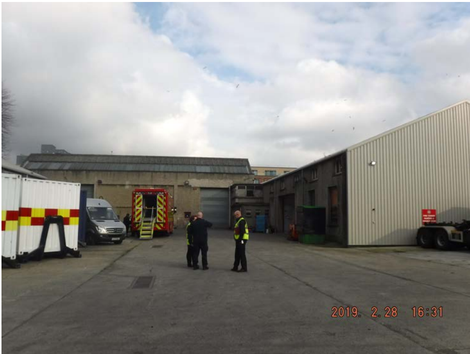
Plate No. 27. General view showing the west elevation to Building No.01.
