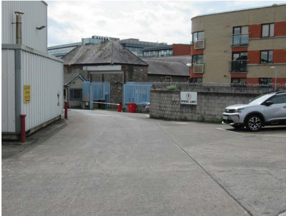
Plate No. 37. General view looking south-east, showing concrete block site boundary wall along the west end of the south boundary. This wall has no architectural or historical significance.
