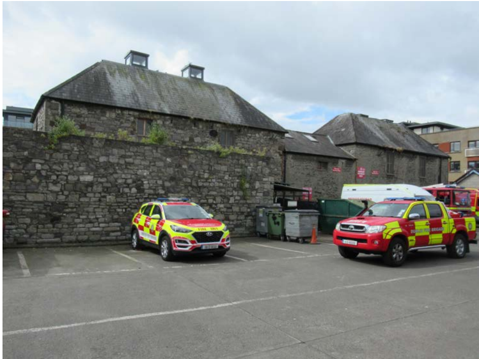
Plate No. 11. Rear north elevation of the former Malting House, showing the characteristic roof forms over the drying kilns, required to dry out the freshly malted barley, to prevent it from continuing to grow. This elevation will continue to be visible from within the proposed development. The length of limestone rubble masonry behind the red and yellow car is the remaining south wall of the L-shaped single storey structure that was part of the Scavenging Depot.
