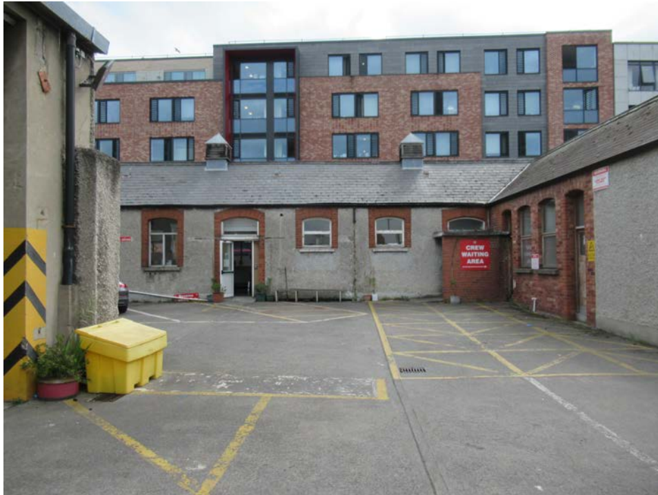
Plate No. 19. General view looking east from within the depot, showing the south-east corner of the L-shaped building in its reduced size. The doors and windows were detailed the same as the openings on the east elevation, as shown in the previous photo.
