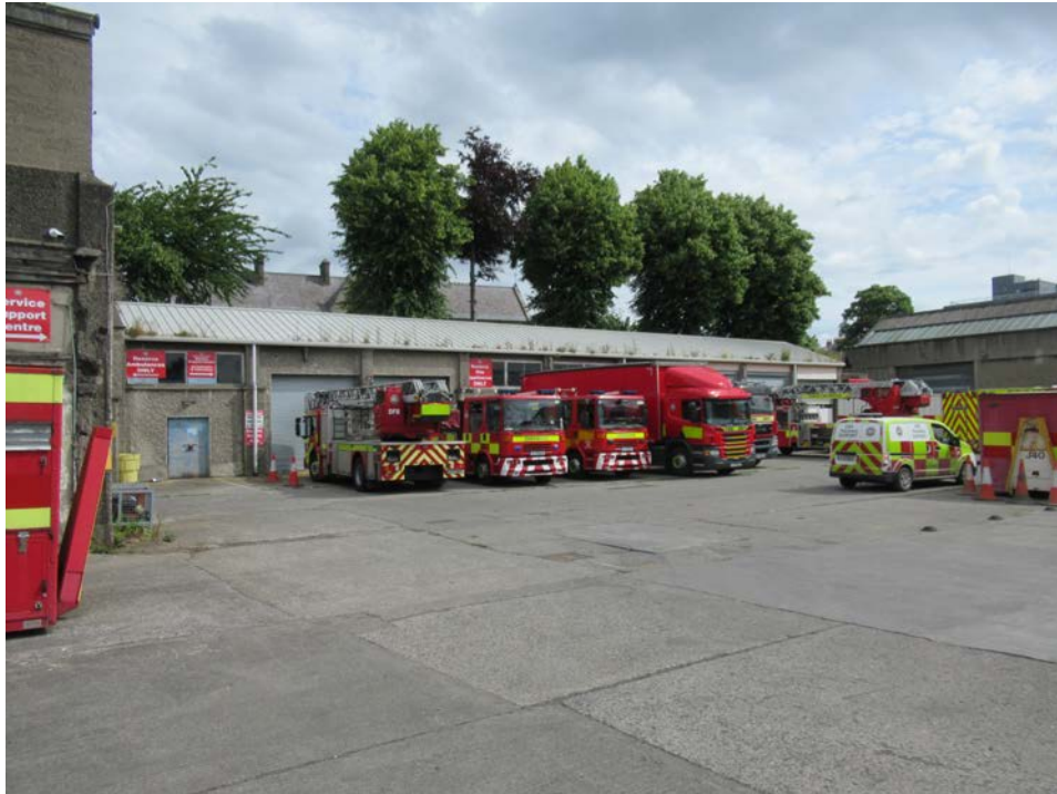
Plate No. 36. General view looking north, showing the repair shops and stores along the northern boundary to the development site, referred to as Building No. 07. This structure dates from the late 20 th or early 21 st century, and were built to serve the Fire Services Dept. None of these structures have any architectural or historical significance and their demolition for the new development will have no negative impact of the historic setting of any protected or otherwise significant structures.
