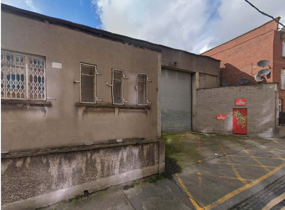
Plate No. 26. General view looking west along Grangegorman Lower, showing Building No. 01, the large storage depot that forms the north-east corner to the current depot. This simple industrial structure is shown on the 1970s OS map, showing that it was in place by at least 1972.
