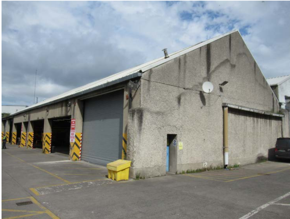
Plate No. 28. General view looking north-west showing the south and east elevations to Building No.5, the main repair garage in the centre of the depot. This structure appears to date largely from the early years of the 21 st century, and stands in the location of the original 19 th century main Scavenging Depot structure. It has a large open plan internally and has minimal architectural or historic significance. The thickness of the east gable wall shown above, and the outline of a smaller gabled building suggests that at least some of the fabric from the late 19 th century depot structure has remained in place. To the rear of this structure, just visible to the right of the gable, are two other long narrow structures that appear to contain fabric from earlier 20 th century building periods, now covered with modern metal cladding.
