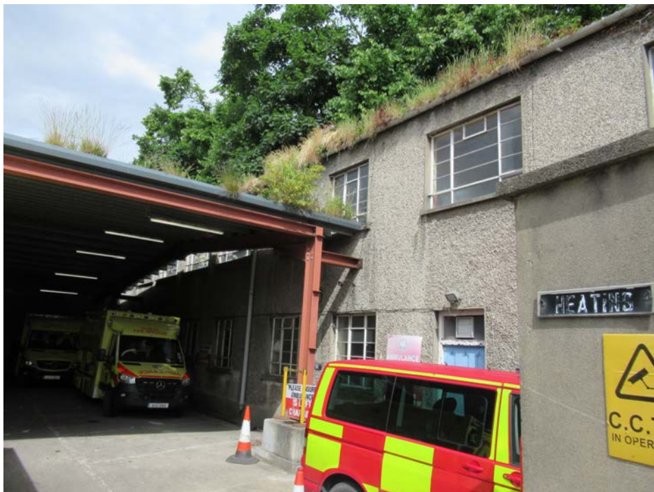
Plate No. 35. General view looking north-west showing the poorly maintained range of offices that forms the northern perimeter to the depot. This structure was shown in the early 20 th century OS map, as surveyed in 1936. The steel framed windows are notable in their design, but are generally representative of typical commercial construction of the time.
