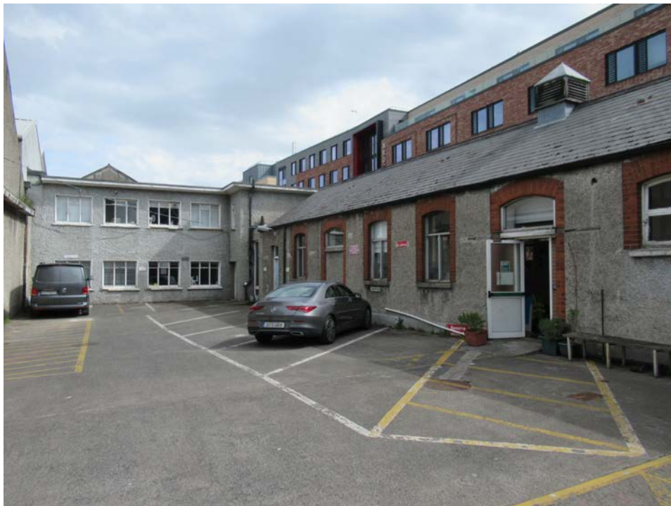
Plate No. 20. General view looking north-east, showing the east range of the L-shaped building in its current reduced form. There are no historic doors or windows remaining in the structure and the stone masonry on the elevations facing into the depot are covered with dashed render.
