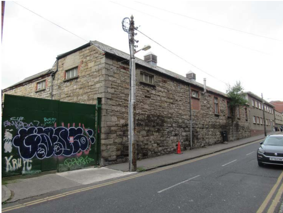
Plate No. 17. General view showing the south-east corner of the 19 th century L-shaped structure and its relationship to Grangegorman Lower. The gate at the left blocks the former entrance to Fountain Place, now in private ownership. Note the massive limestone quoins in the corner, compared to the finer grain of the coursed rubble masonry on the rest of the walls.
