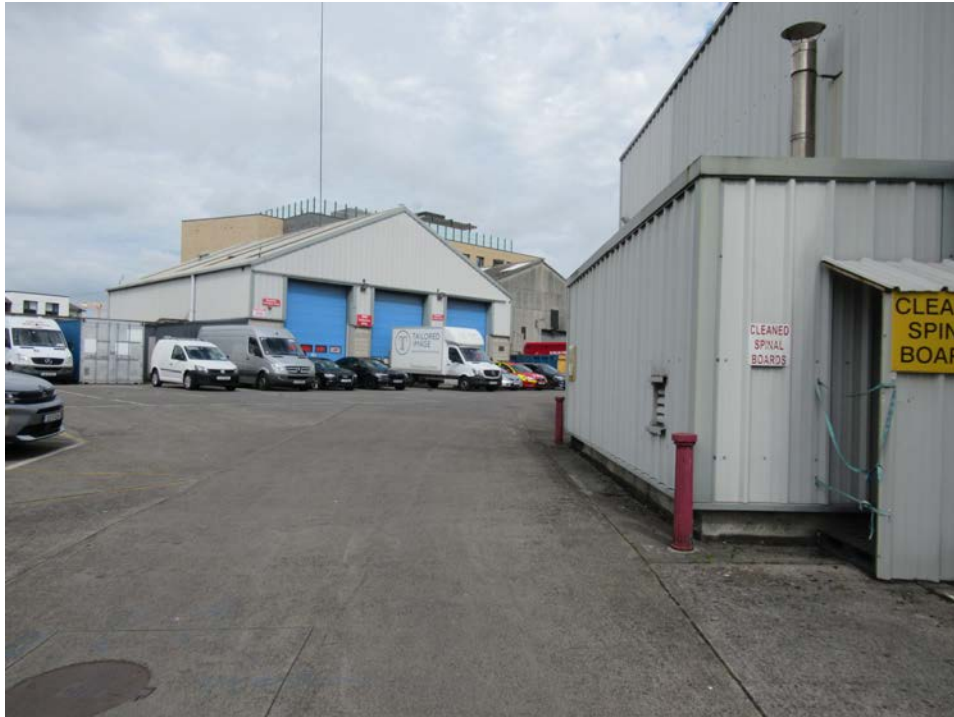
Plate No. 31. General view looking west across the depot, showing Building No. 6, a medium sized steel clad garage for storing emergency vehicles. This structure dates from the early 21 st century and has no particular architectural or historical significance.
