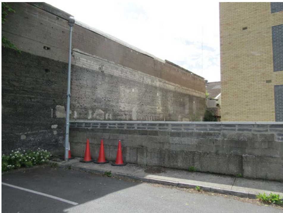
Plate No. 42. General view looking south-east, showing same cast concrete site boundary wall at the north-west corner of the development site, as it appears from the adjacent school car park. It is proposed to retain this wall, because it is now a party structure, but to reduce its height as part of the demolition of the 20 th century industrial structures in the north-west corner of the development site.
