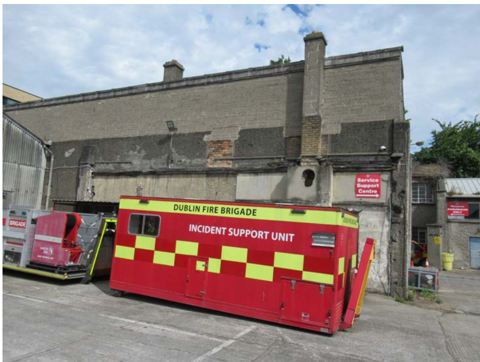
Plate No. 33. General view looking north the rear of the south range of Building No.04. The following photos show the other elevations to that early 20 th century range of structures.
