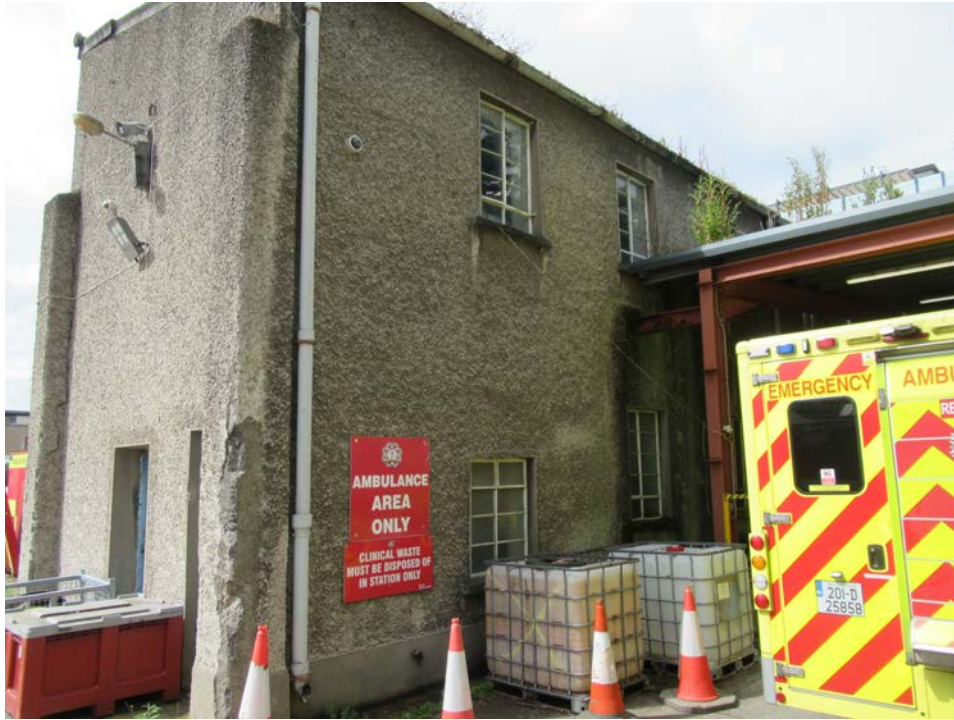
Plate No. 34. General view showing the north elevation of Building No. 04, the Scavenging Depot structure from the previous photo. This is a simple utilitarian structure of the 1930s without any particular architectural or historical significance. This structures in this photo and the following photo are shown in the north-west corner of the Scavenging Depot in the OS map shown in Plate No.6, showing the area in 1936.
