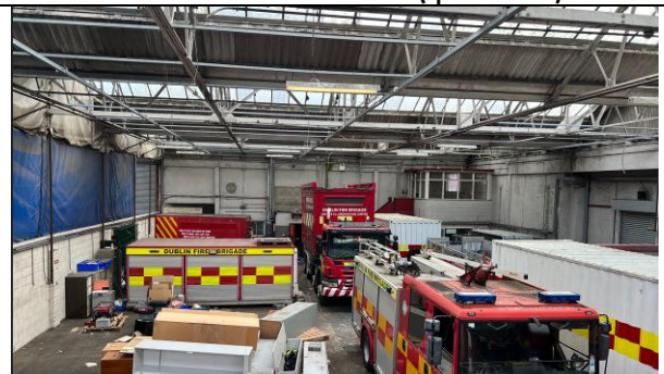
Internal Side view ( photo 26)
