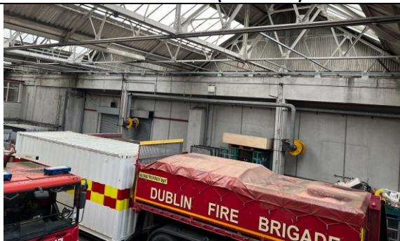
Internal Side view ( photo 25 )
