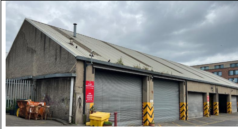
Roof view external side ( photo 45)
