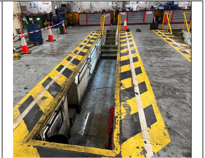
Internal view ground floor slab (Photo 42)
