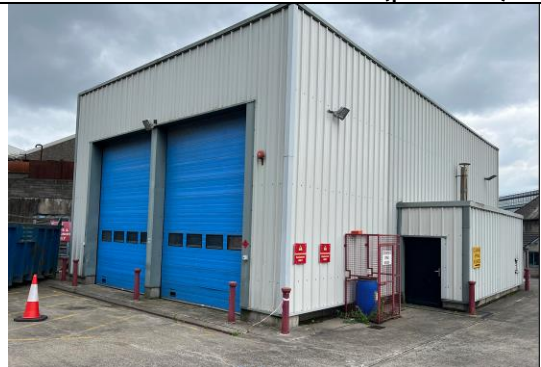
External View - rear side (photo 22)
