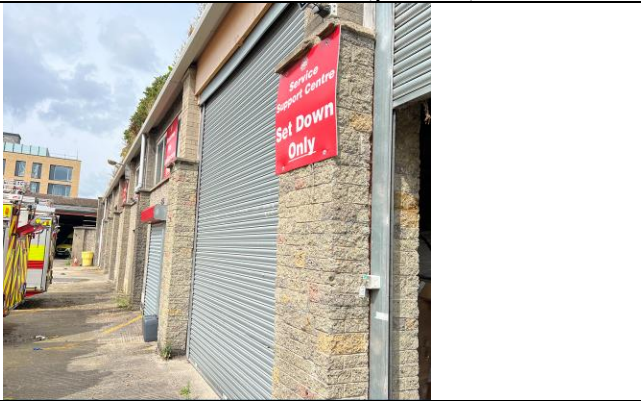
External View (photo 10)
