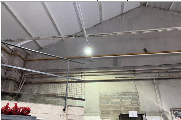
Internal Side view ( photo 31 )
