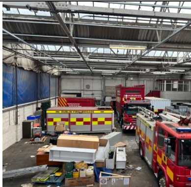
Internal View (Photo 23)
