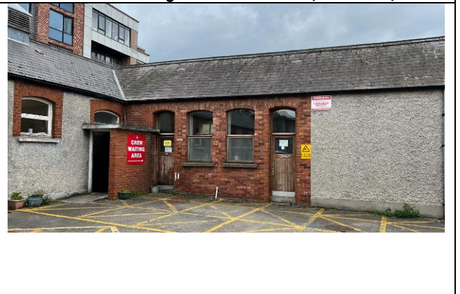
Roof view external side ( photo 50)
