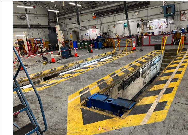
Internal view ground floor slab (Photo 41)
