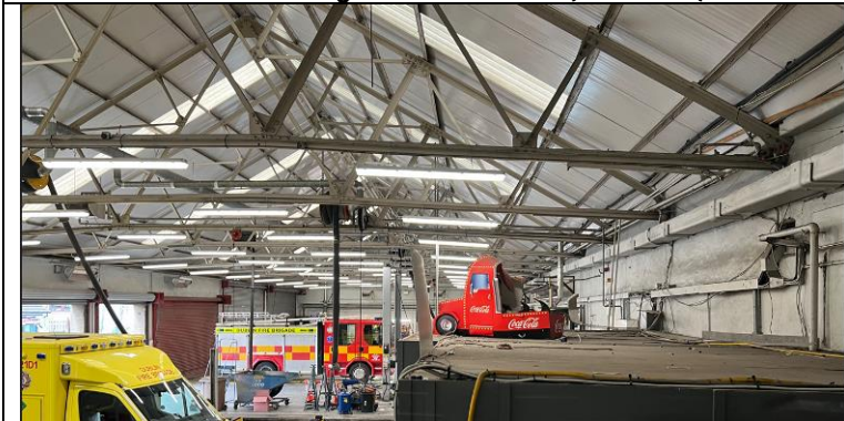
Roof view ( photo 43 )
