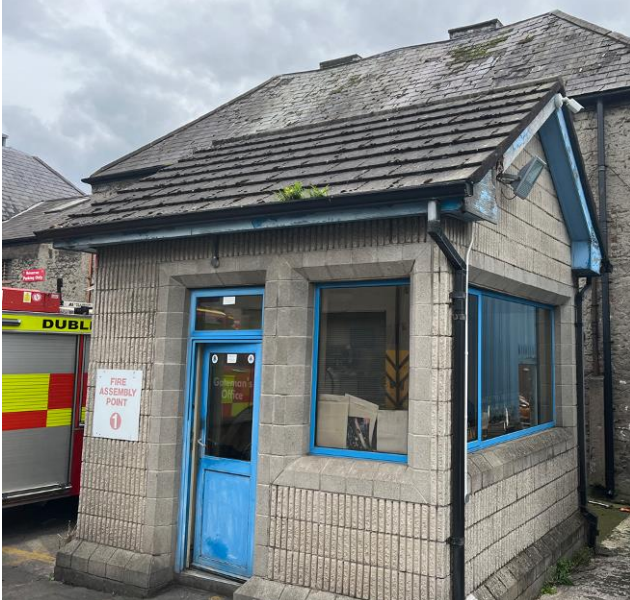
External view (Photo 58)
