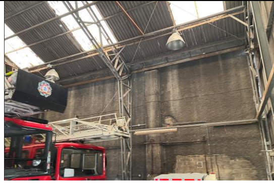
Internal view – external wall, Right side (photo 14)
