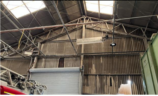
Internal view – front elevation of the building (photo 13)
