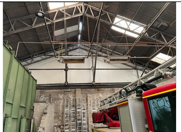
Internal view - roof structure (photo 12)
