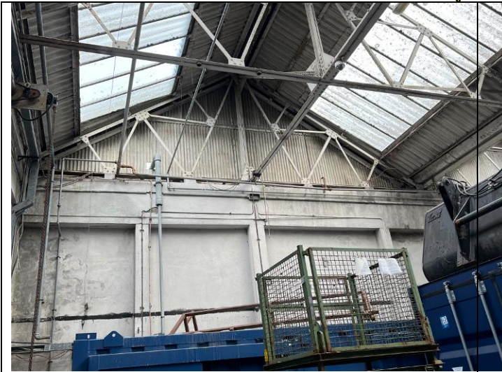
Roof view (photo 27)
