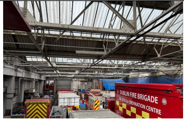
Internal view -rear side ( photo 24)
