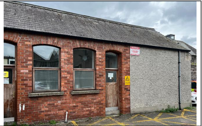
Standard Internal side of the building (photo 52)
