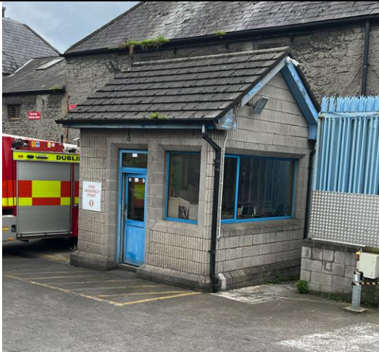
External view (Photo 56)
