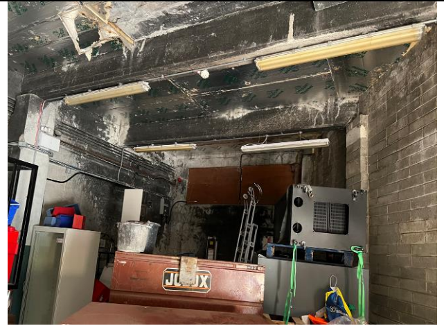
Internal view - standard room (photo 8)
