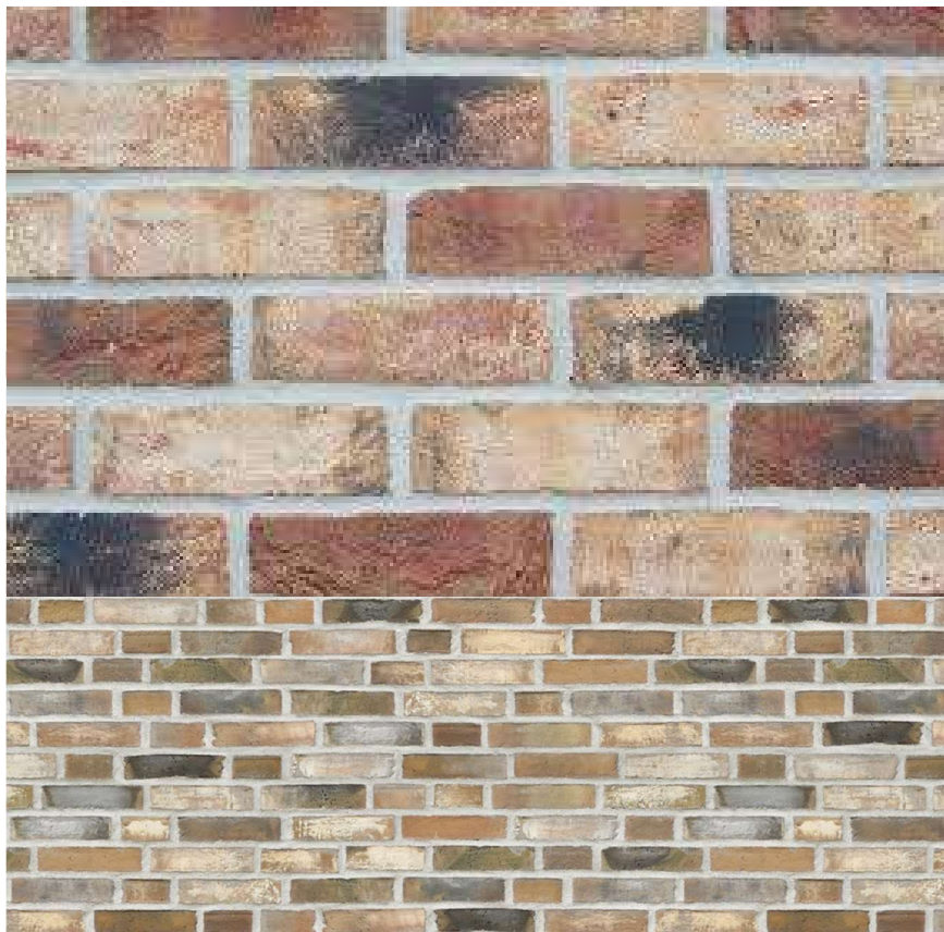
Figure 33. New development to be clay multi brick – buff base with reds and burnt blends to tie-in with tones in the local area.
