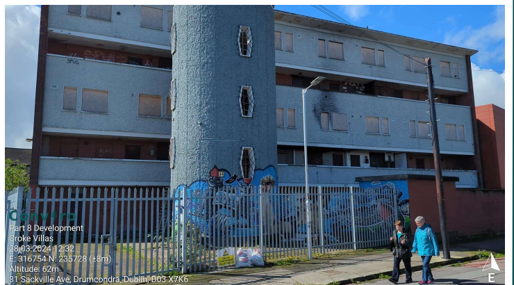
Photo 4: Croke Villas flats requiring demolition. .
