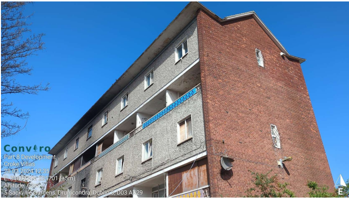
Photo 5: Rear of Croke Villas flats requiring demolition.
