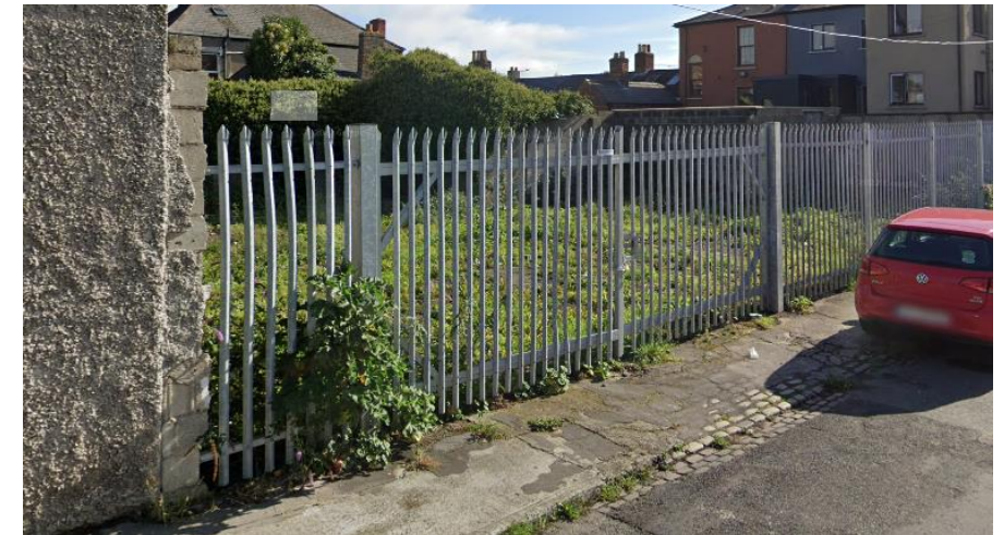
Figure 36: existing palisade fence to north side of Sackville Avenue
