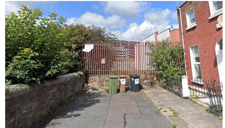
Figure 37: existing palisade fence and wall removed and bollard provided
