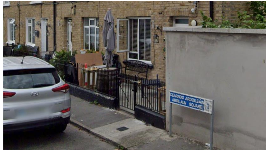
Figure 33: existing lows walls and railings to Ardilaun Square retained.
