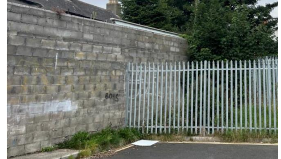
Figure 35: existing walls to rear of Sackville Gardens retained and rendered to public realm
