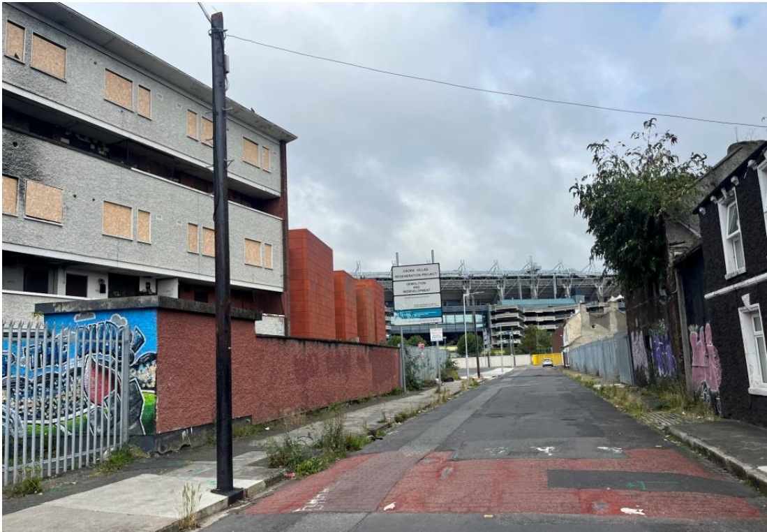
Photo 1: View of the existing building to be demolished along Sackville Avenue.
