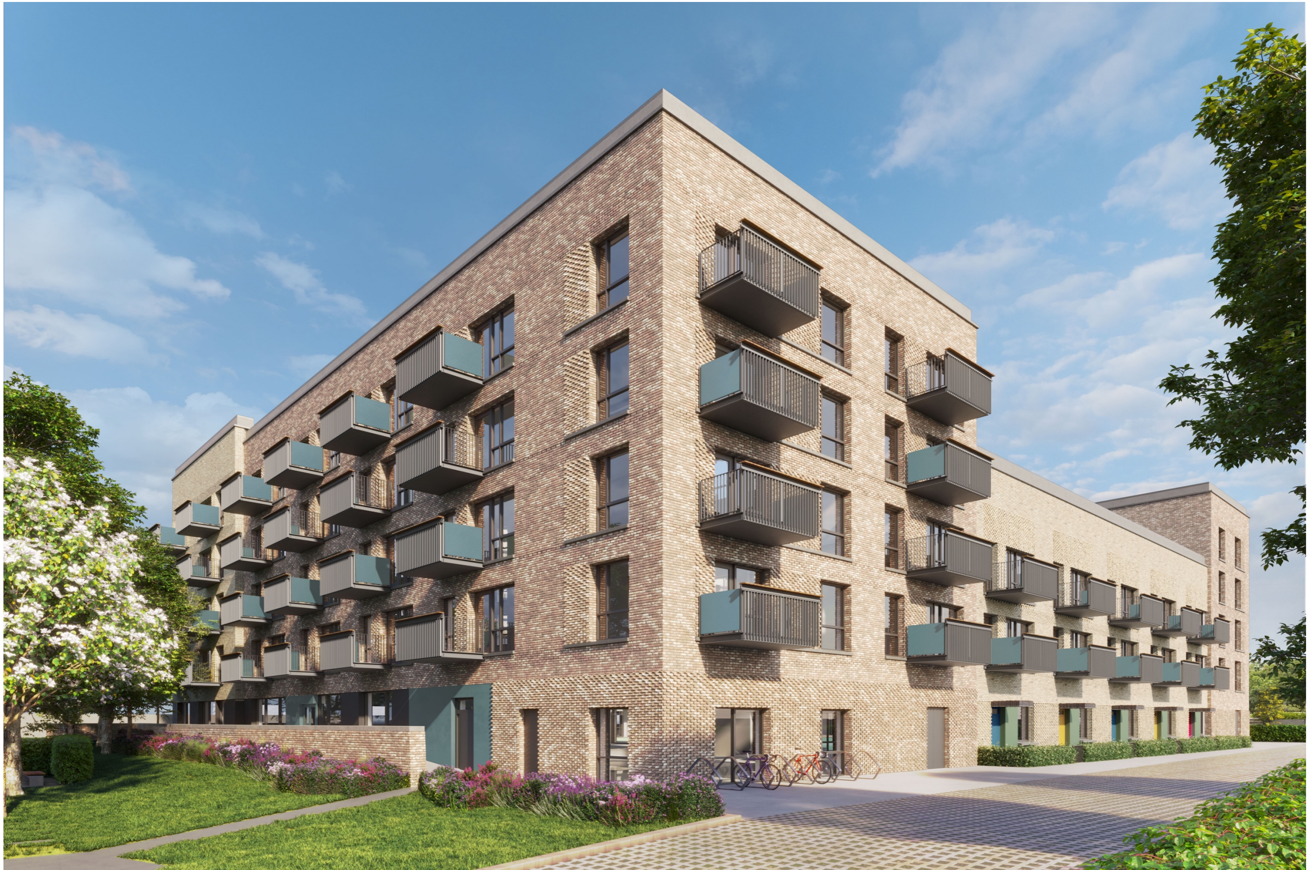
04 – View Looking North-East
