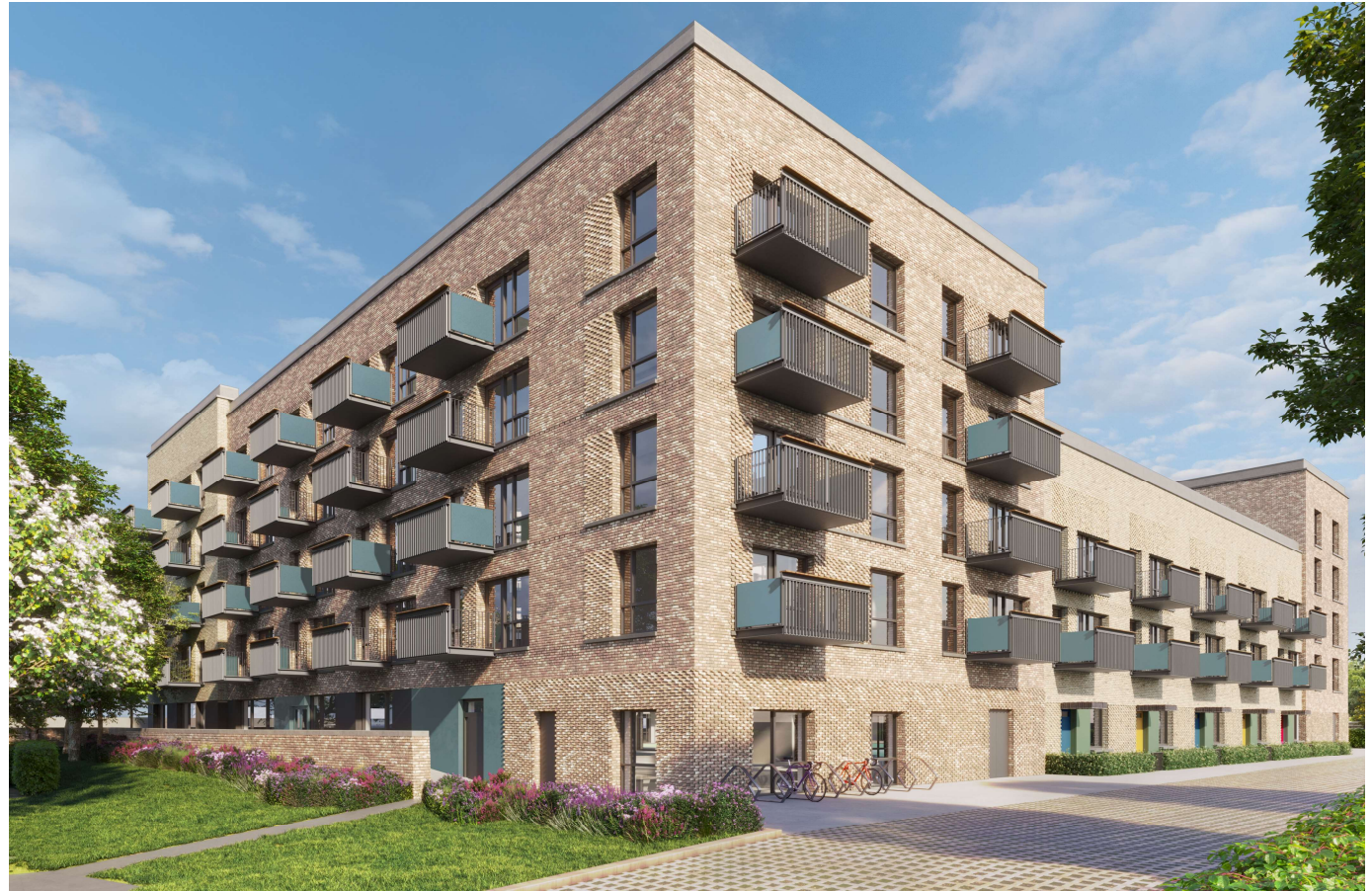
Above: View Looking South West
