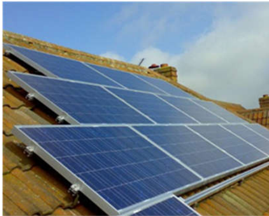
Typical Photovoltaic Arrangement
