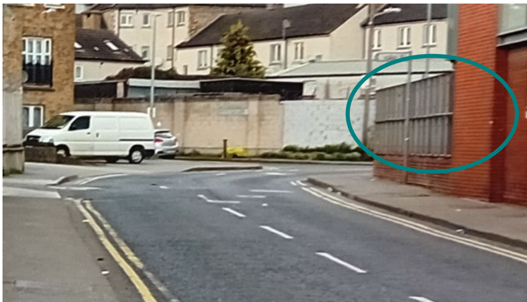
Figure 6.3 – Existing boundary wall and railing
