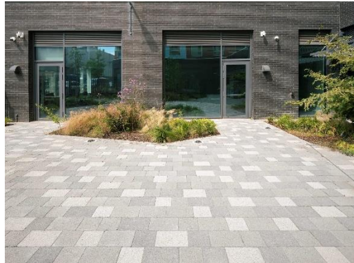
Example of mix colour pavers for amenity courtyard Reference pictures taken from Tobermore catalogue
