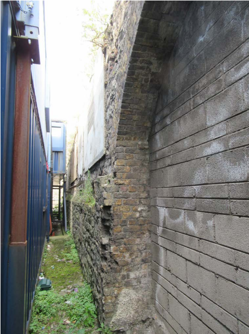
Plate No. 36. Detail view looking west along the inside of the northern boundary to the depot, showing the brick lining to the historic arched gate onto Forbes Lane, currently infilled with concrete block.
