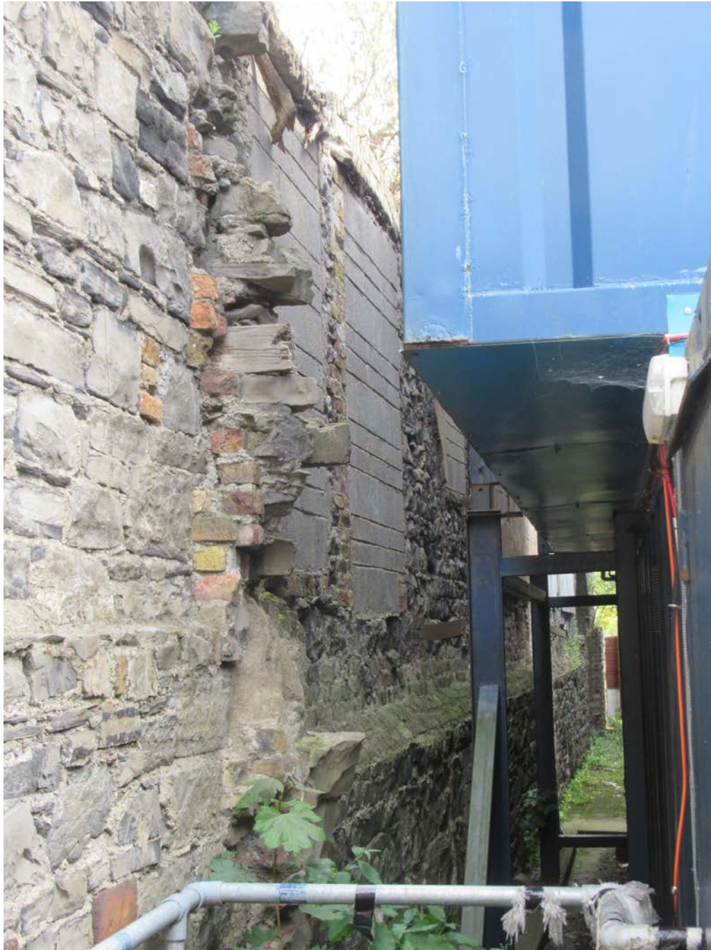
Plate No. 34. General view looking east along the northern edge of the depot site, showing the south side of the stone boundary wall. The concrete blocks are filling in the window openings that can be seen on the other side of the wall, where a section of 19 th century masonry survives from one of the distillery buildings along Forbes Lane. This section of wall, with infilled window ope and an invilled arched gate, is proposed for retention as a fragment of the distillery, in the proposed development.
