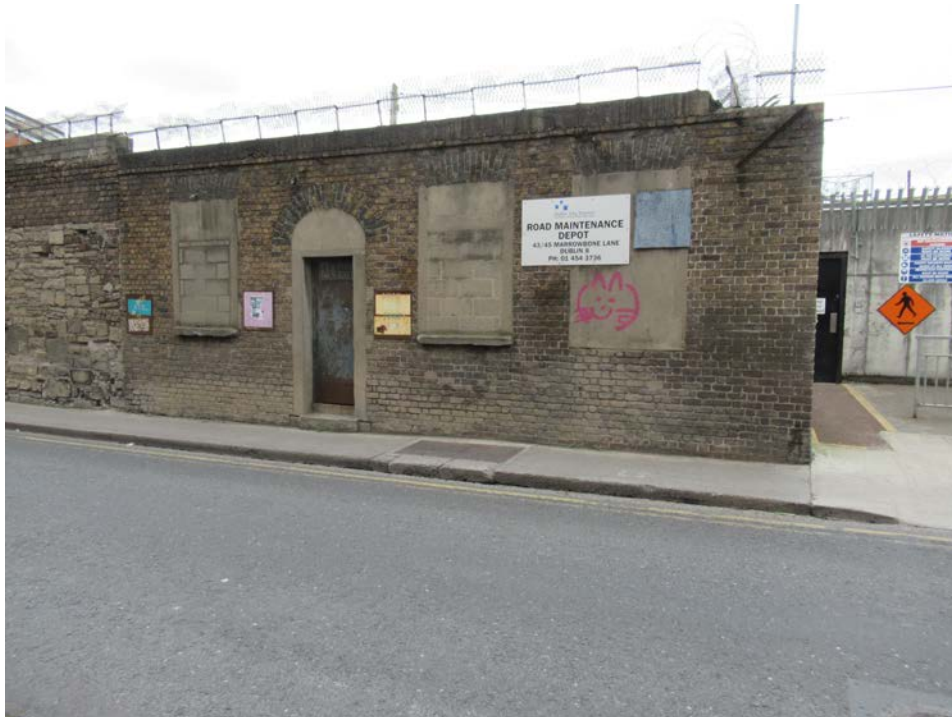
Plate No. 27. General view looking west, showing the surviving east elevation to the historic structure that stood at the entrance gate to the distillery. This structure is shown on the 19 th century illustration of the distillery.
