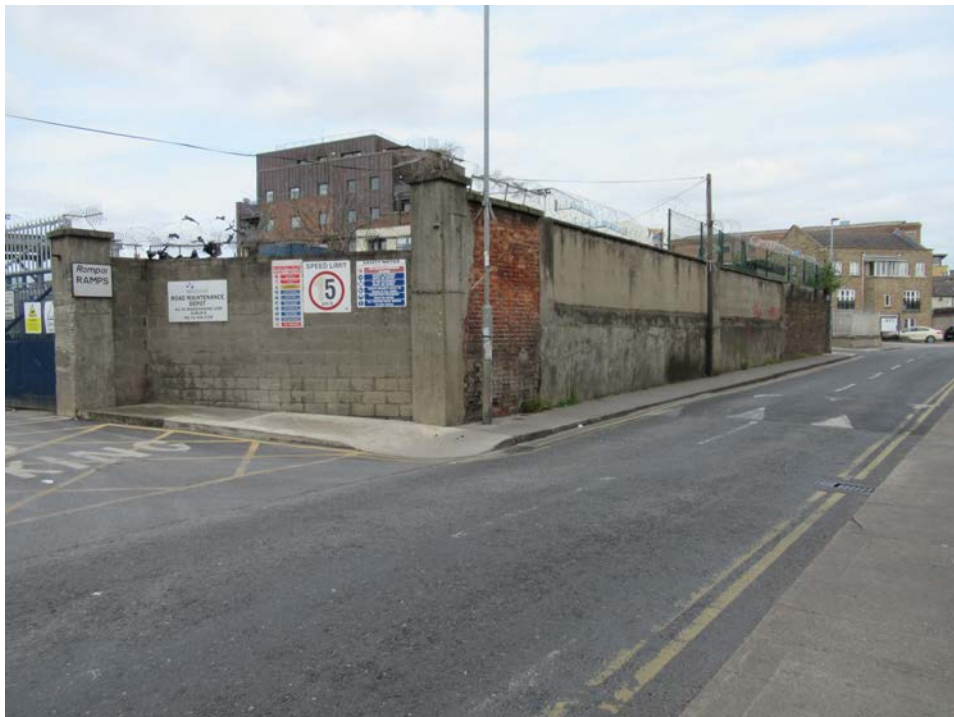
Plate No. 26. General view looking north-west, showing the norther end of the perimeter wall along Marrowbone Lane.
