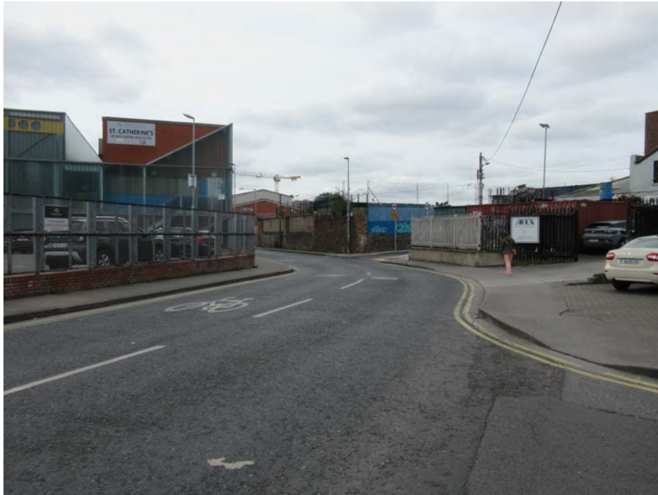
Plate No. 21. General view looking south-west along Marrowbone Lane, towards the north-east corner of the development site. This is the approximate location of the historic photo that shows early 19 th century gabled houses on both sides of Marrowbone Lane, with the distillery chimney in the background.
