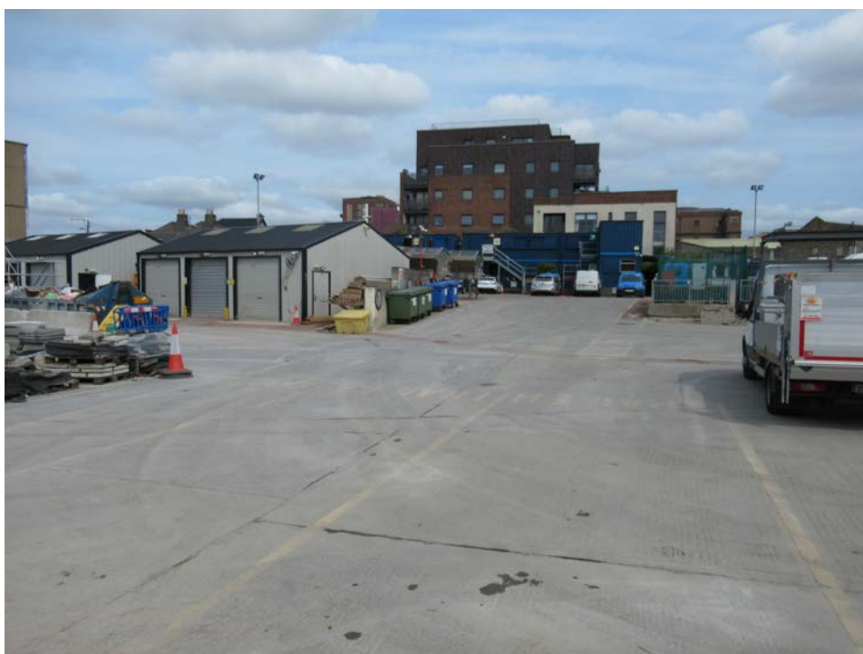
Plate No. 32. General view looking north across the depot site, showing the range of light industrial structure dating from the late 20 th and early 21 st centuries. None of these structures have any architectural or social significance.
