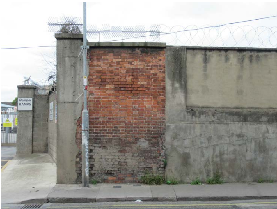
Plate No. 24. General view looking west showing the north side of the entrance gate into the current depot, with a small section of good quality 19 th century red brick masonry surviving from the distillery.
