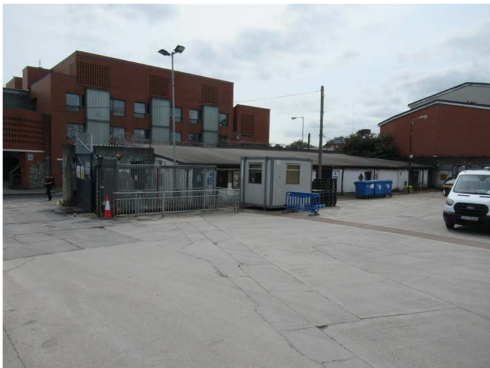
Plate No. 38. General view looking south-east across the depot, showing the main entrance into the depot at left, with the community centre structure on the east side of Marrowbone Lane is seen behind the wall. The row of store rooms with the single pitched roof dates from the late 20 th century, and is built against the inside of the old masonry perimeter wall on Marrowbone Lane.
