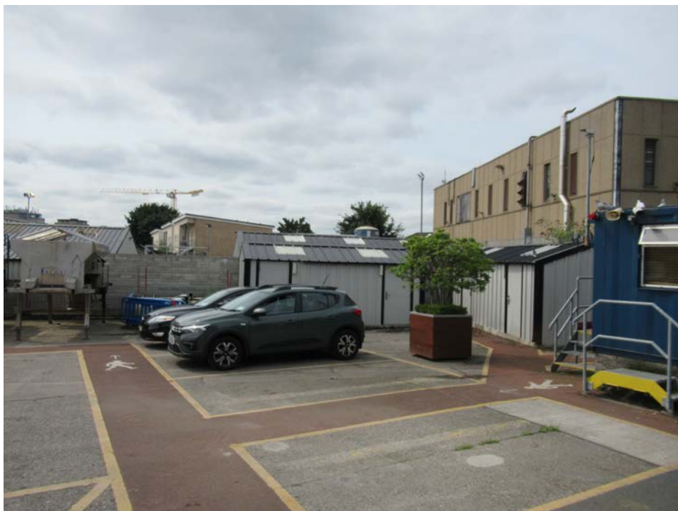
Plate No. 31. General view looking north-west across the depot site, showing the porta-cabin structures that house staff offices, toilets and break rooms. The two store structure is the telecommunications complex in the adjacent site.
