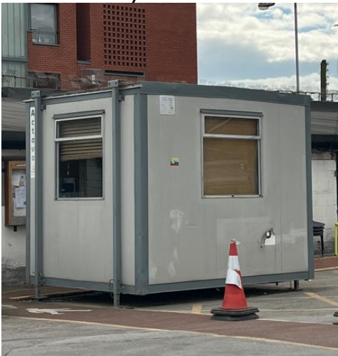
Modular Security cabin.
