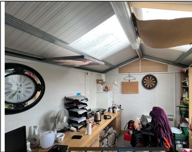
internal view - Photo 13
