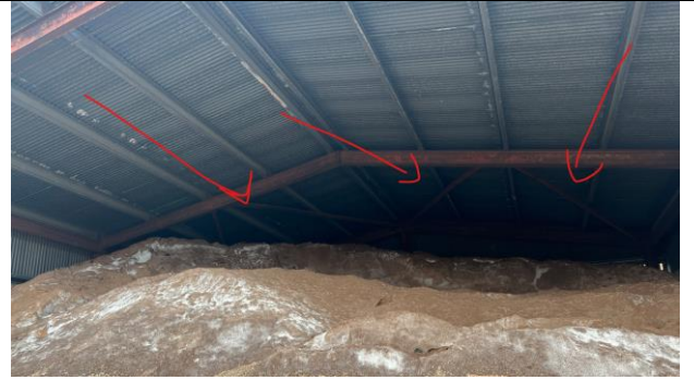
Top view- rear bracing - Photo 2
