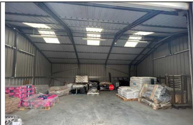
Concrete floor - Photo 24
