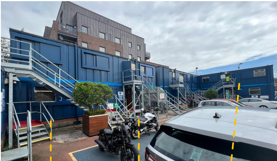
Porta cabine 1 With 2 levels
