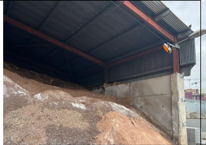
internal side - First Floor - Photo 4
