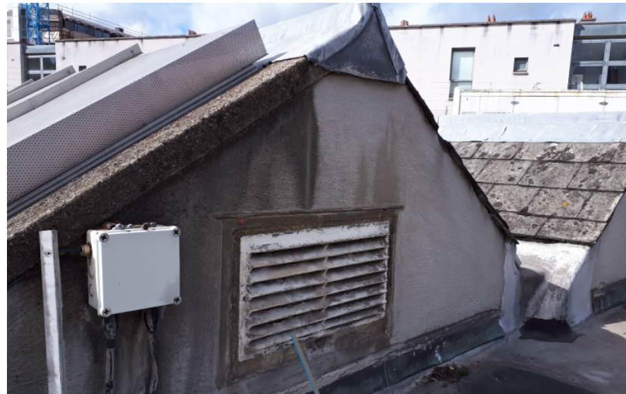
Existing Vents To be Utilised where possible
