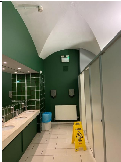
Fig 21. North wall of room no.22.B1.005.
