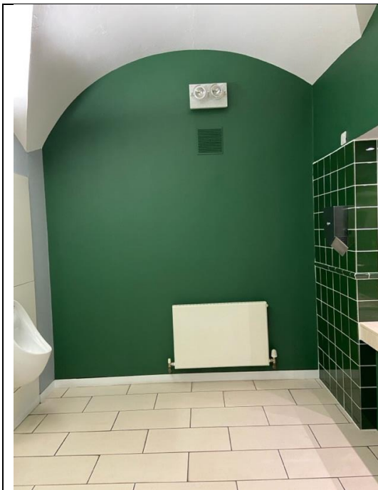
Fig 20. North wall of room no.22.B1.004.
