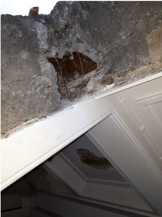
Existing concrete encased beams to be exposed
