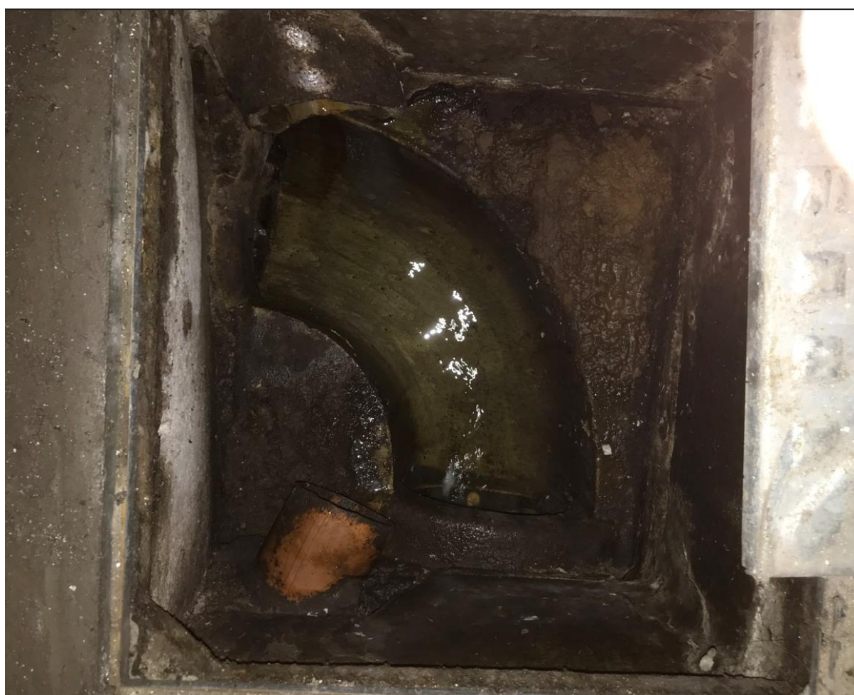
Figure 5. Existing Drainage outfall Manhole within Hugh Lane Gallery Basement (Source: AECOM).
