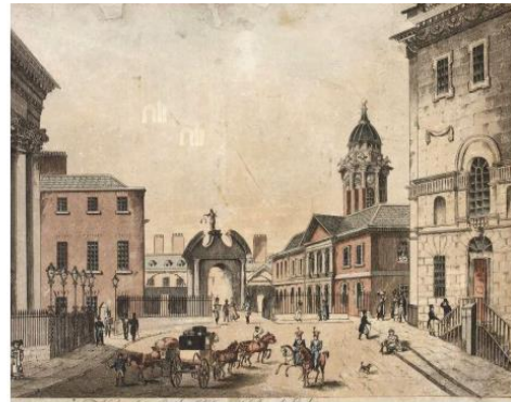
View of the Castle Gate and Royal Exchange 1810-1858 Henry Brocas, Source NLJ
