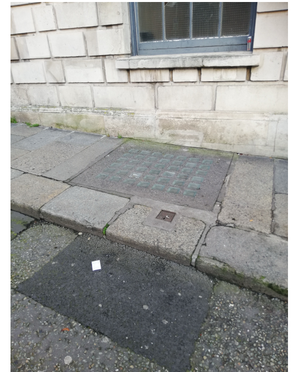
Existing concrete pavement light.
