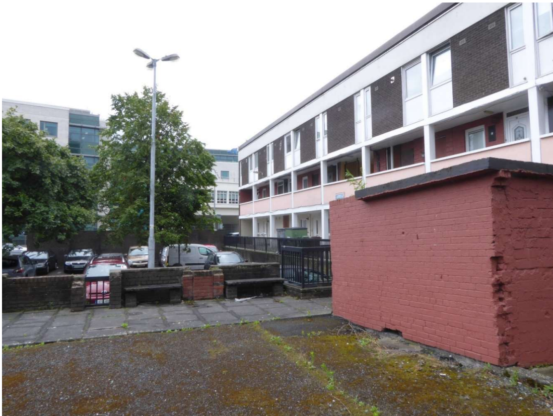
Figure 2 Site showing building and trees in carpark.
