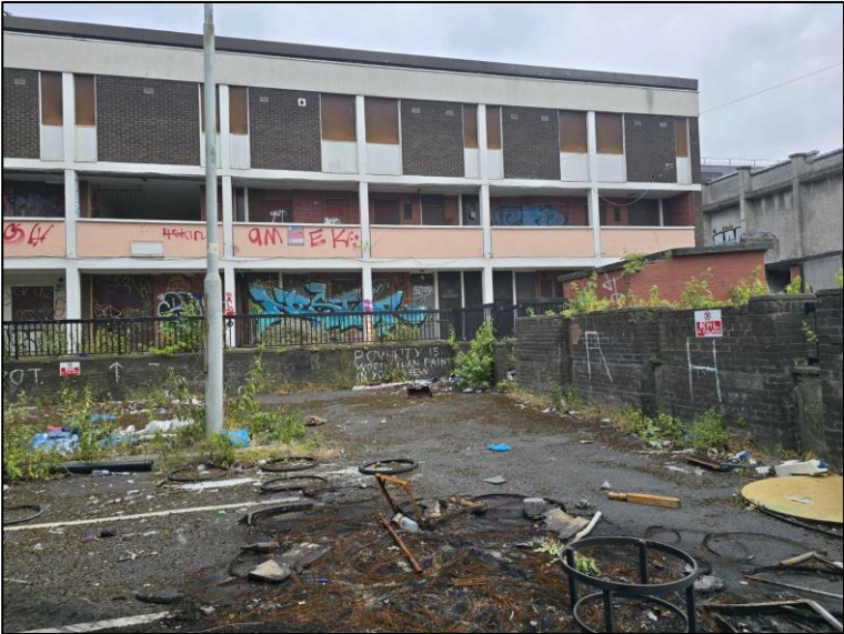
Plate 3 Rear of affected structure located within Dublin city area with Negligible Bat Roost Potential.
