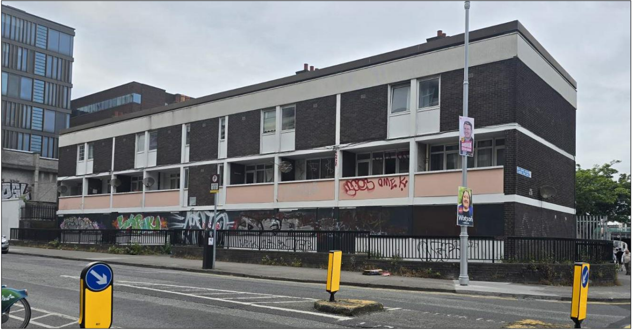
Plate 1 Front of affected structure within city area with Negligible Bat Roost Potential.
