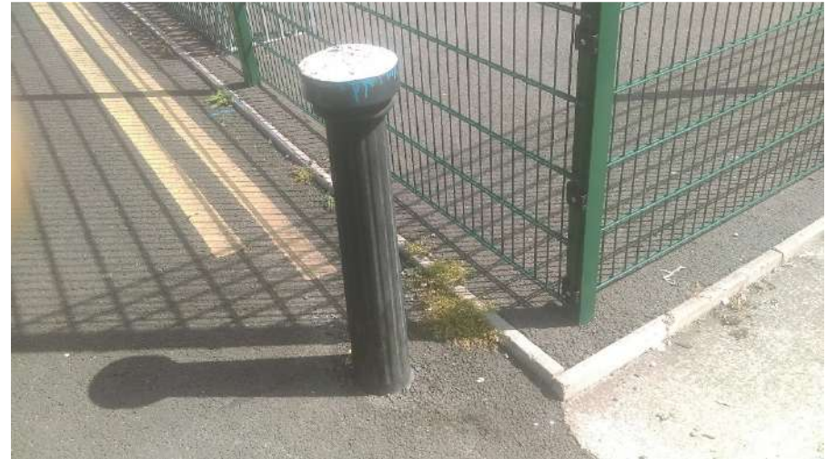
Plate 10 Bollard at southwest corner of playground, facing northeast
