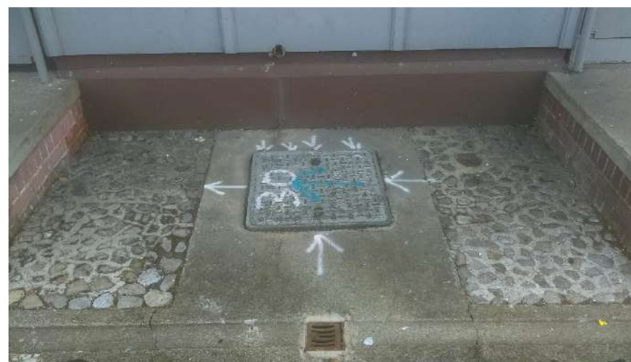
Plate 4 One of manholes along front of the ground floor bedsits with cobbling, facing southeast
