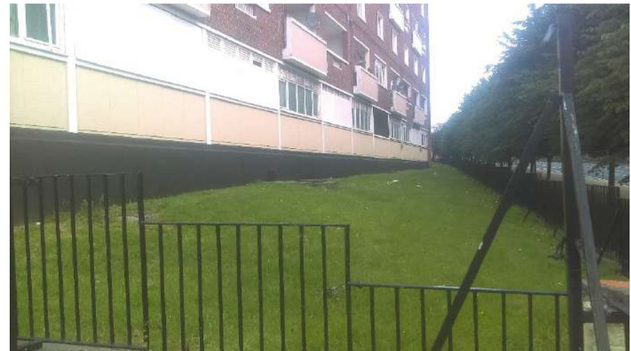
Plate 8 Back (eastern side) of southern building along Constitution Hill, facing north
