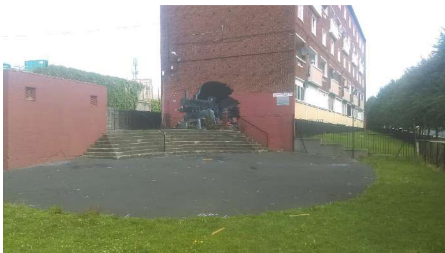
Plate 3 Southern end of southern building, facing north
