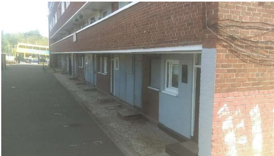
Plate 7 Front (western side) of northern building, facing northeast
