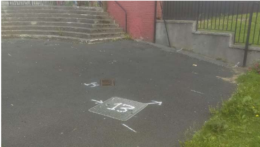
Plate 5 Manhole and drain in southern tarmacked area, facing northwest
