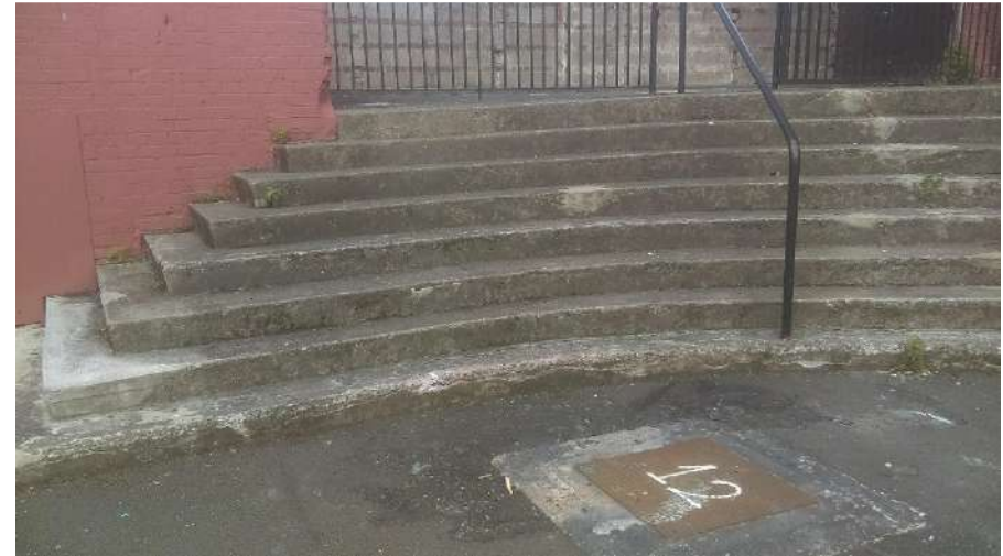
Plate 6 Manhole at base of steps. Southern tarmacked area. Facing northwest
